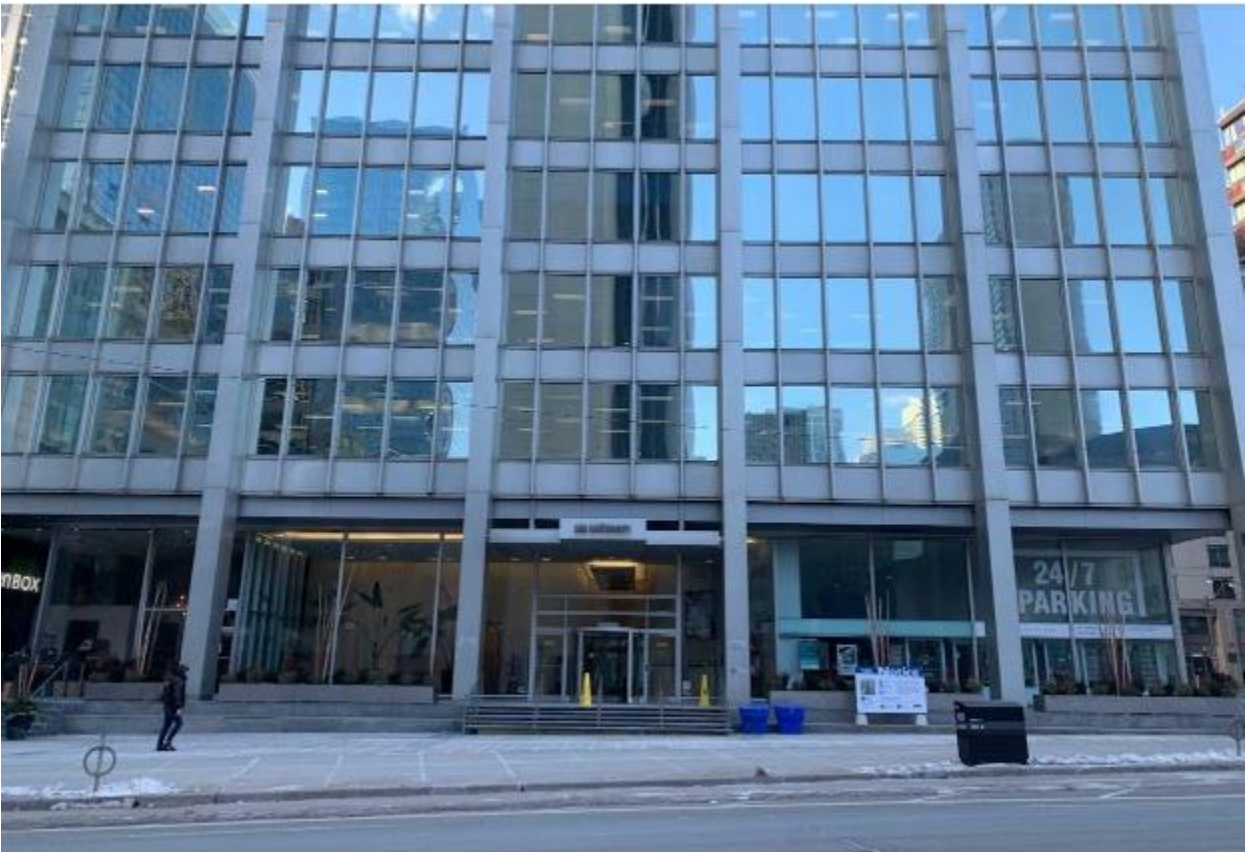
View of the east elevation with glass-clad ground floor and mezzanine level and the metal-clad perimeter columns (ERA, 2022)
