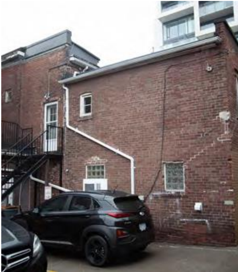
Figure 12 2111 Yonge Street south elevation (ERA Architects Inc, 2023).
