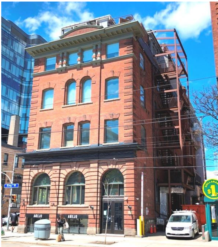
Photograph of the principal (south) façade on King Street West and the side (east) facades on the laneway. (HP, 2021)
