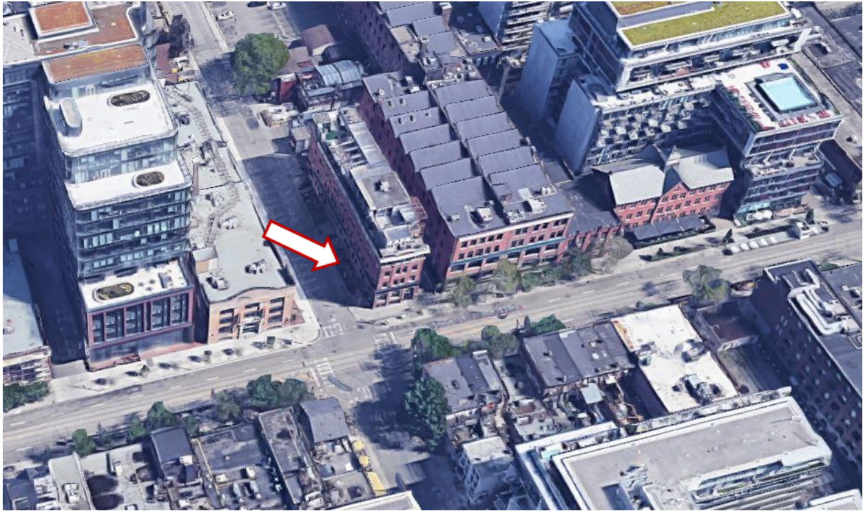
Aerial view of the subject property at 600 King Street West at the north-east corner of King Street West and Portland Street. (Google Maps, 2021)
