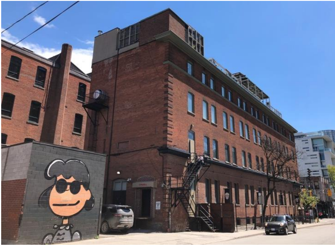
Photograph of the north side of the property showing the one-storey outbuilding that is proposed to be demolished and the rear façade of the Beatty Manufacturing Company Building. (HP, 2021)
