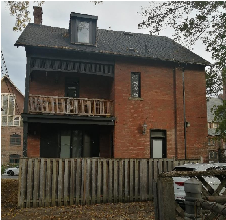
Figure 10 South (rear) elevation (Heritage Planning, 2023).
