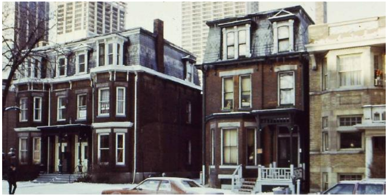
Figure 5: 1974 image showing 66 Charles Street East and adjacent properties (Toronto Historical Board).
