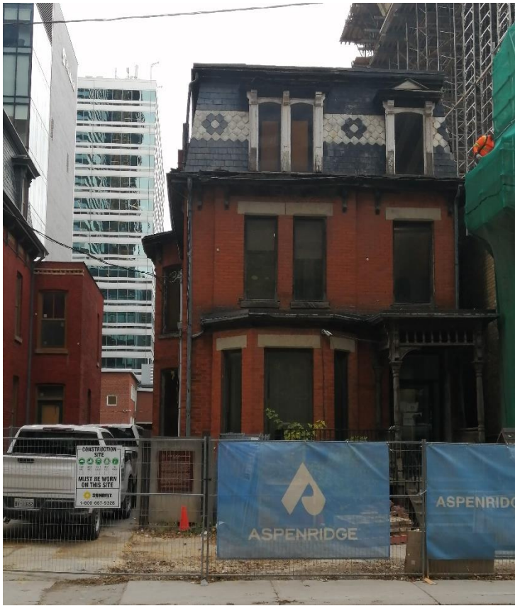
Figure 6: Principal (south) elevation of 66 Charles Street East (Heritage Planning, 2023).
