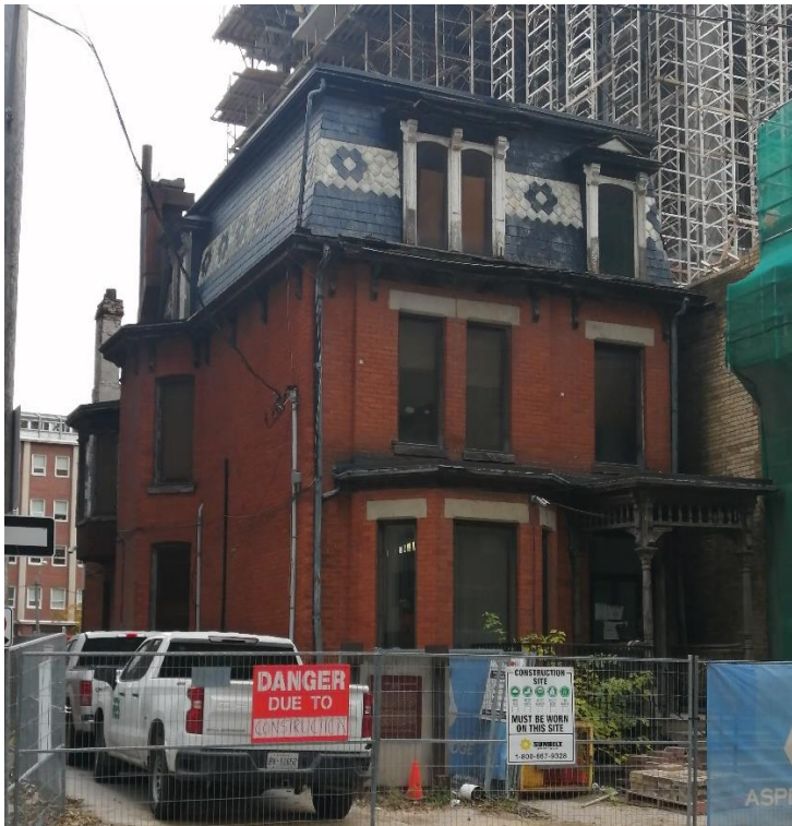
Figure 7: South and west elevations of 66 Charles Street East (Heritage Planning, 2023).
