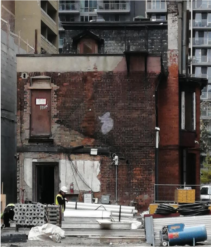
Figure 8: Rear (north) elevation of 66 Charles Street East (Heritage Planning, 2023).
