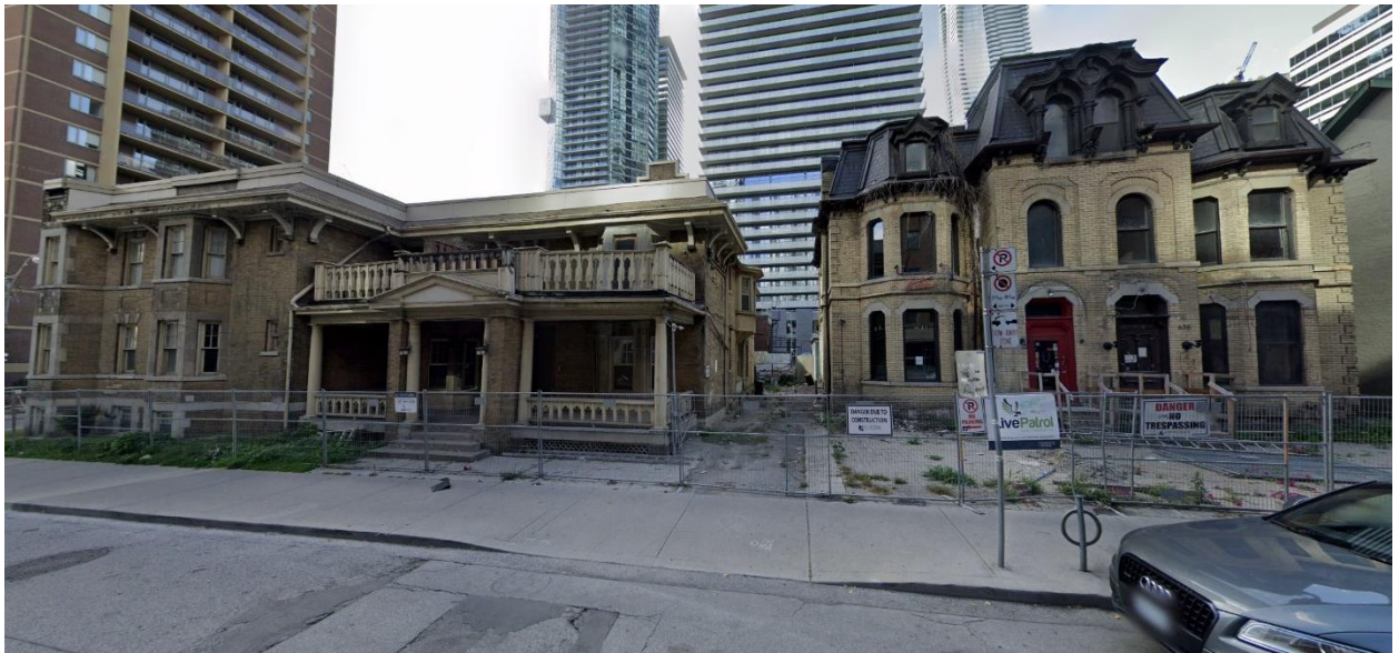
Figure 11: 2019 image looking west towards the Part IV Designated properties at 628 Church Street (left) and 634-636 Church Street (right). The current views of 628 Church Street and 634-636 Church Street are obscured by scaffolding as part of their inclusion in a high-rise development (Google Streetview).
