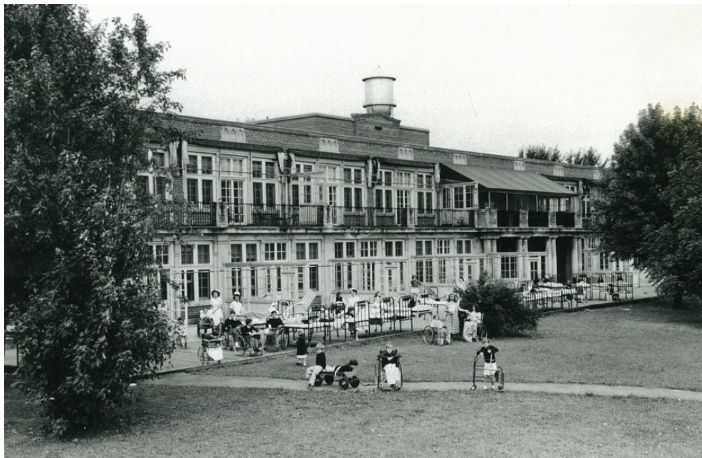
25. Image of south elevation of the patient wing with children and staff, with beds rolled out onto the boardwalk. The south elevation was purposefully designed and constructed for heliotherapy, n.d. (Hospital Archives, The Hospital for Sick Children)
