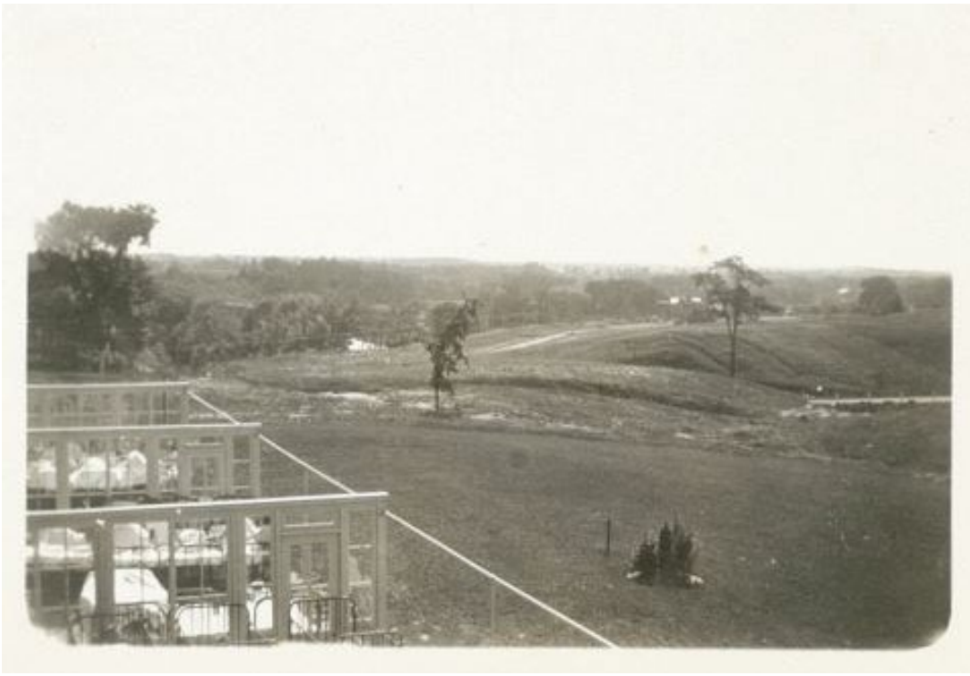
18. View from the second level of the south elevation of the patient wing showing a view to the southeast of the entry road from Islington Avenue with the Humber River beyond. Note the landscape's rolling topography, n.d. (Hospital Archives, The Hospital for Sick Children)
