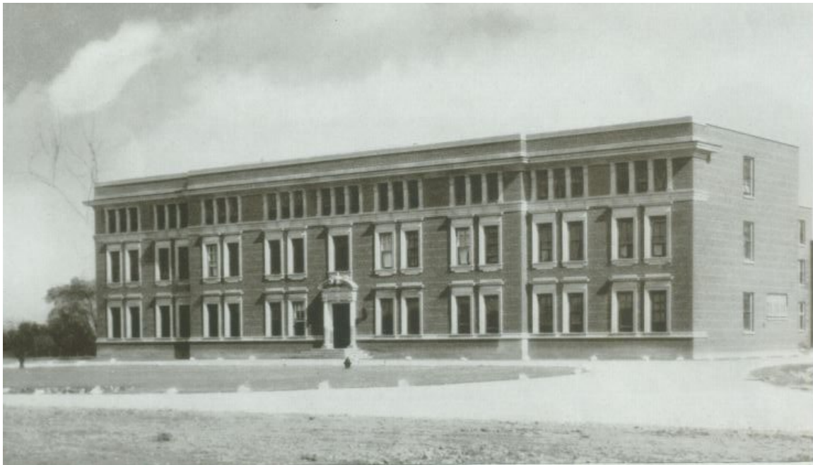
8. Photograph of the building's north façade which was the public face of the building. Note the architectural elements of the Georgian Classical style. (Construction Journal, June 1929)
