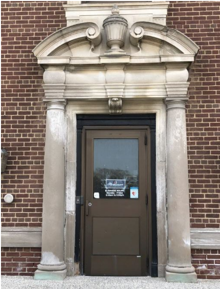
11. North façade, main entrance door with Classical detailing (Heritage Planning, 2022)
