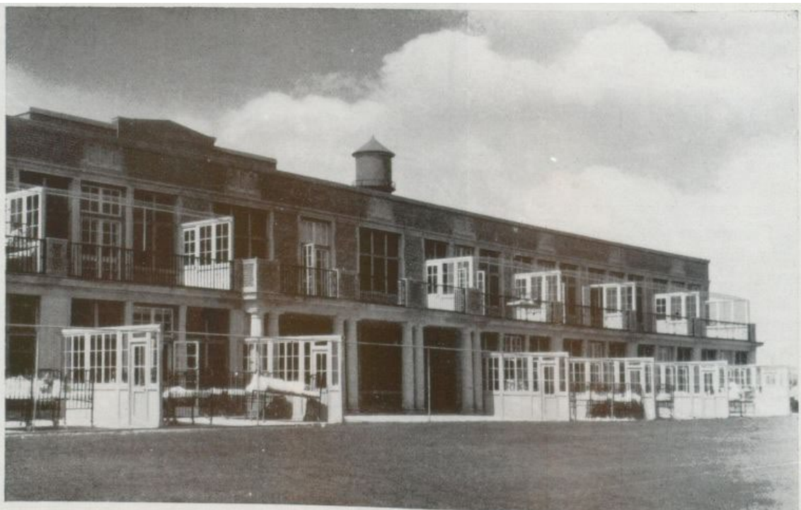
9. Image showing the south façade of the patient wing (south wing) which was specifically designed and constructed for the use of heliotherapy. Doorways permitted beds to be wheeled outside onto wide balconies which extended the entire south elevation. This enabled children to receive direct sunlight and the therapeutic benefits of the nearby pine trees. (Construction Journal, June 1929)
