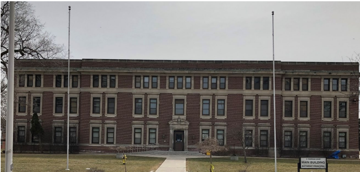
10. North façade was the building's principal public face. It housed the administrative, admissions, and medical facilities. (Heritage Planning, 2022)
