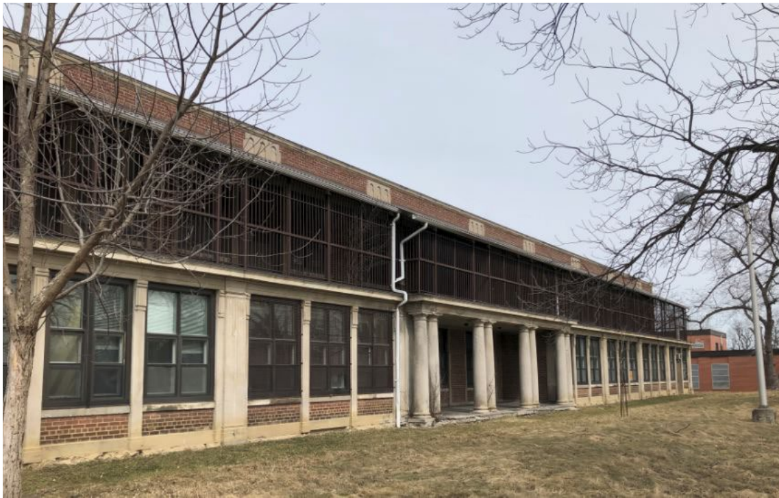
13. South façade with stone details of the central loggia with 4 pairs of Tuscan Doric columns and adjacent pilasters flanking windows. Balconies on the 2nd storey were enclosed in 1959, and in 1990, windows were replaced. (Heritage Planning, 2022)
