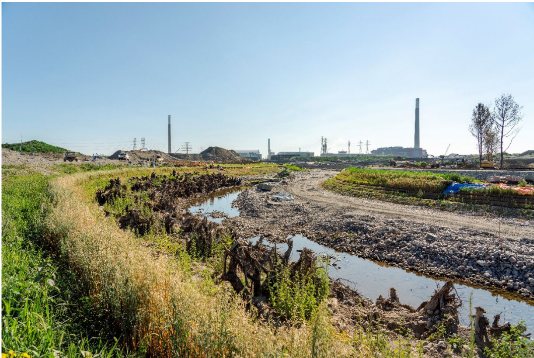
Summer 2022 construction of the new river valley with riverbanks, looking southeast.
