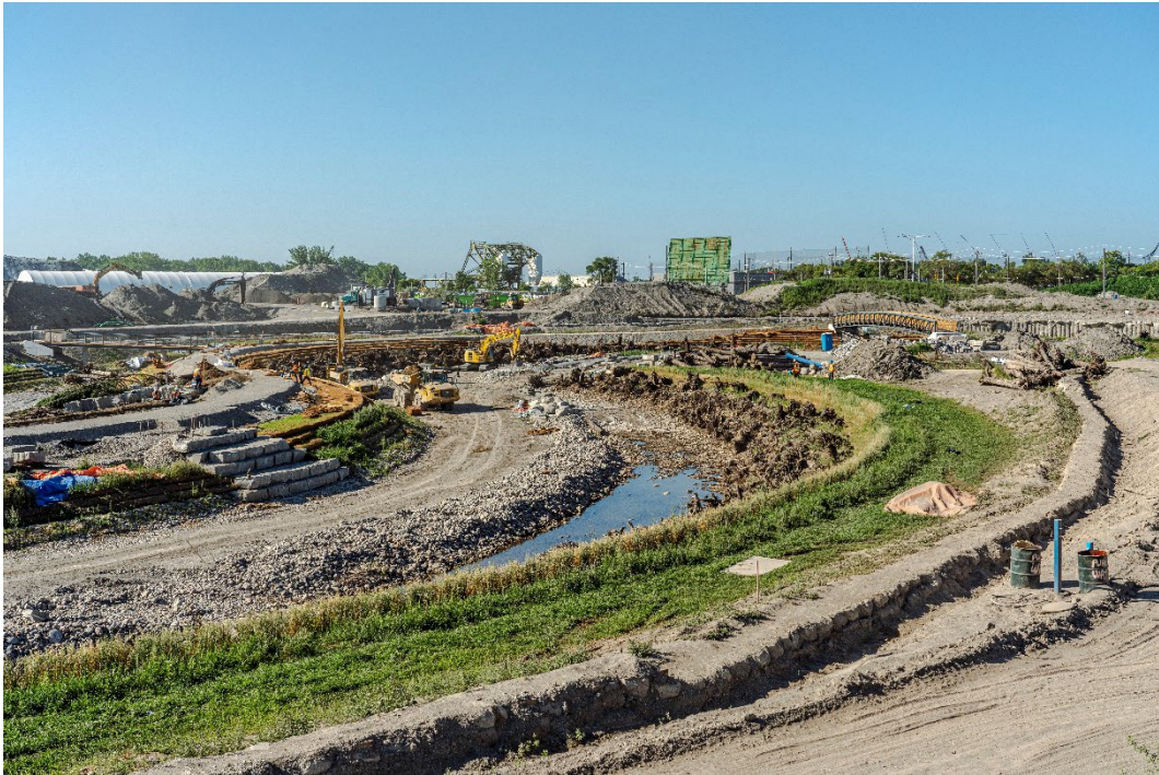
Summer 2022 construction of the new river valley with riverbanks, looking southwest.
