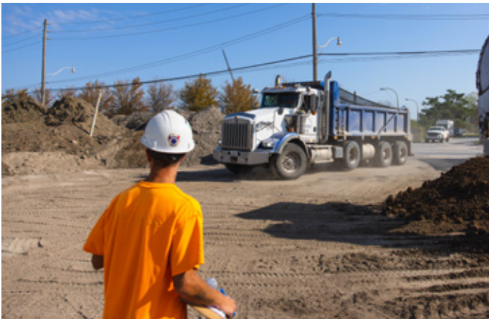
Leslie Lookout Park construction
