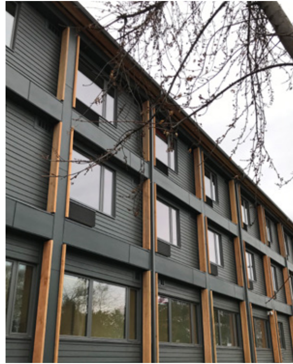
Delivering Modular Housing: 540 Cedarvale Avenue
