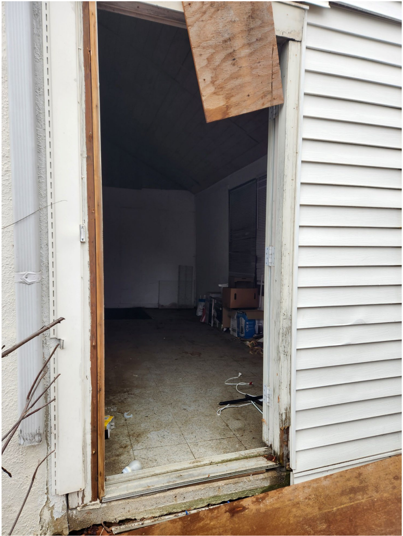
Residential Demolition Application- 14, 18, 24, 26 Jopling Avenue South
