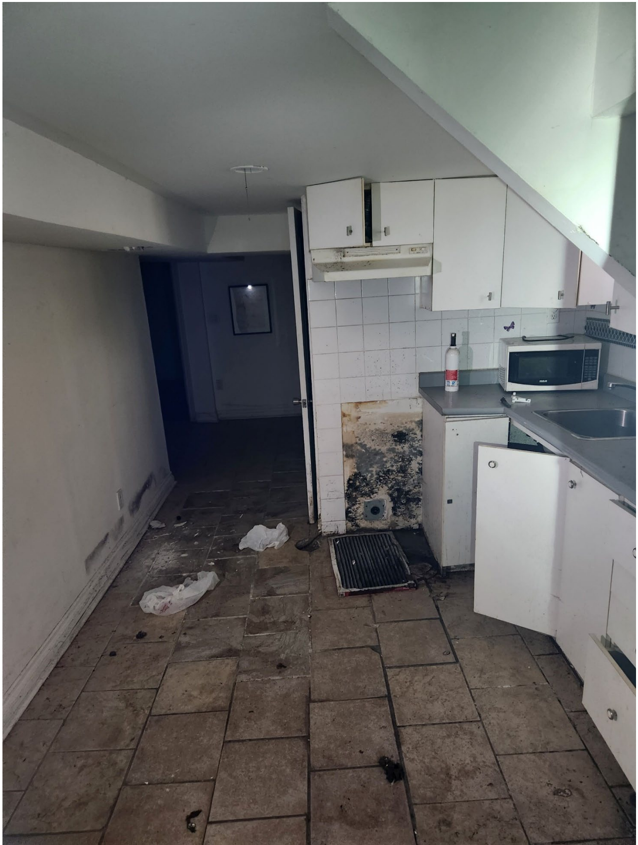
Residential Demolition Application- 14, 18, 24, 26 Jopling Avenue South
