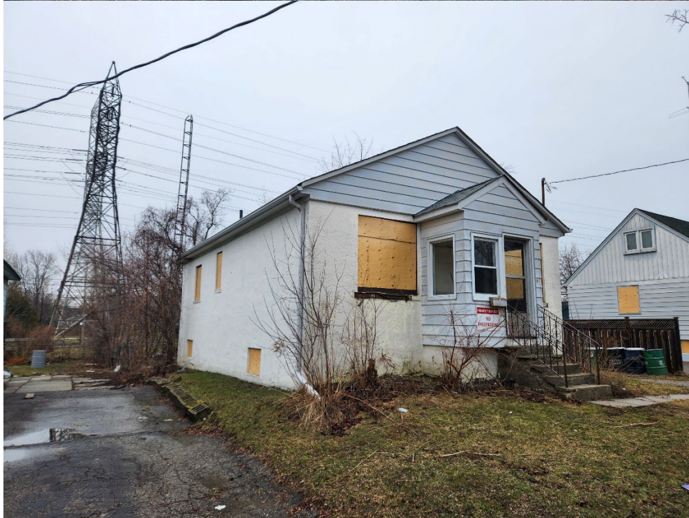
Residential Demolition Application- 14, 18, 24, 26 Jopling Avenue South
