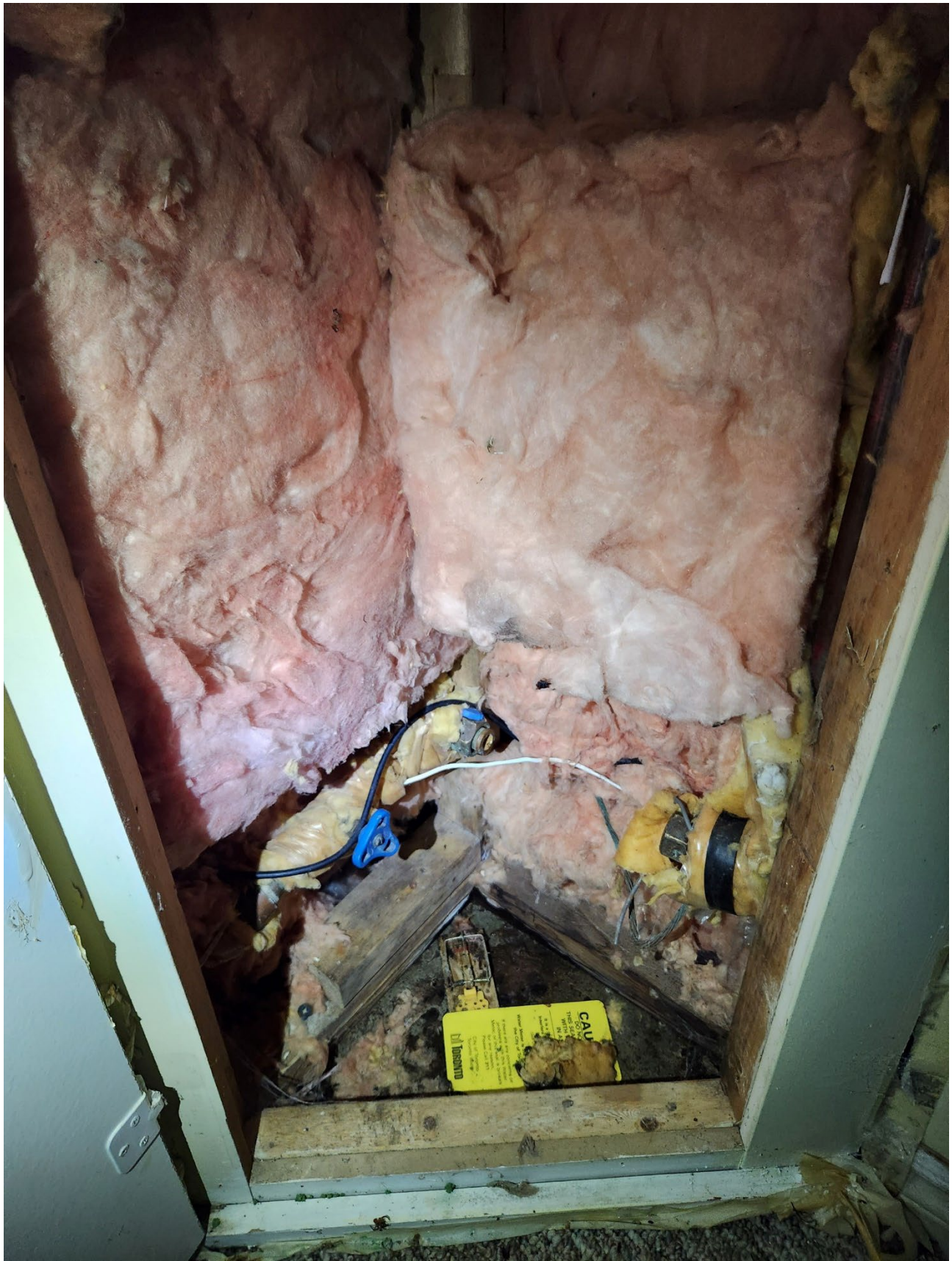
Residential Demolition Application- 14, 18, 24, 26 Jopling Avenue South
