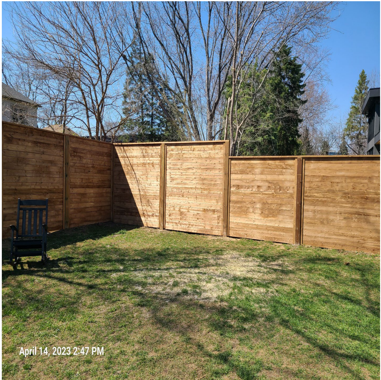
Photo of wood perimeter fence
