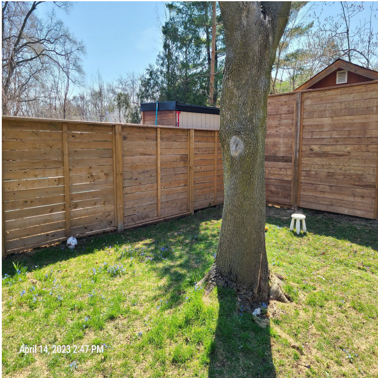
Photo of wood perimeter fence
