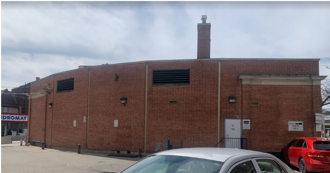
View looking northeast at the rear elevation of the former bank building (Heritage Planning)
