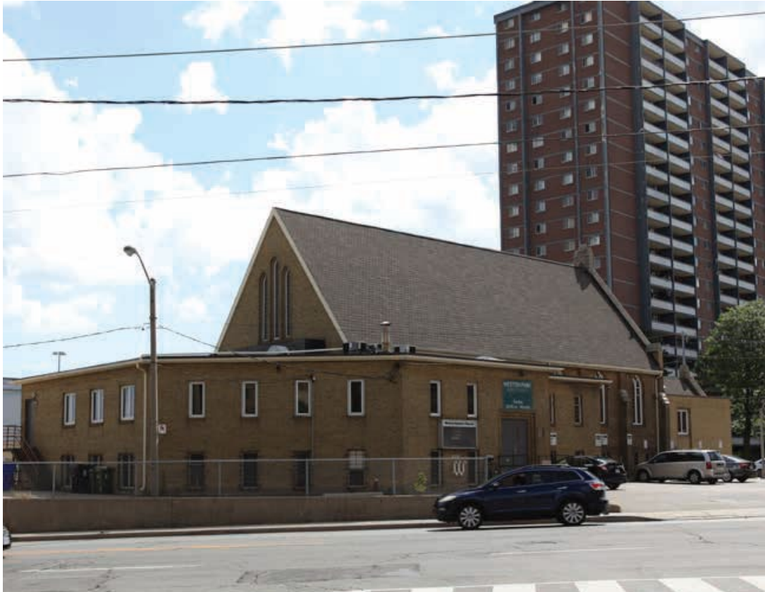
View looking southeast across Lawrence Avenue West at the 1962 rear wing (ERA, 2021)
