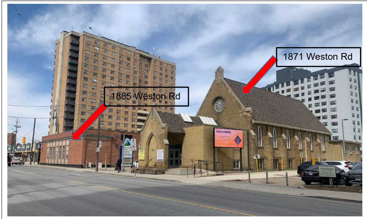
View looking northeast at 1885 Weston Road to the left (former bank building) with 1871 Weston Road (Weston Baptist Church) (Heritage Planning 2023)
