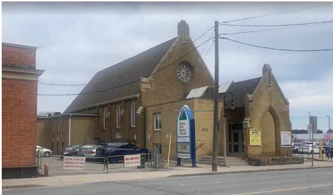
View looking southeast at the north elevation of the nave and 1983-1984 rectangular vestibule fronted by the reconstructed 1947 vestibule façade. Part of the 1962 rear wing is also visible at left (Heritage Planning, 2023)
