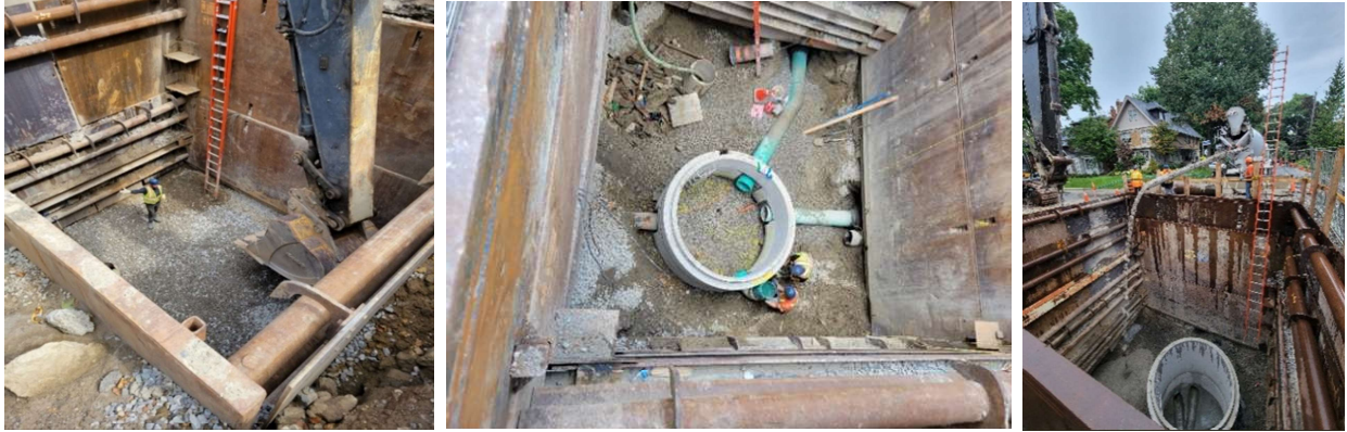
Figure 5 - Drilling Pit on Ridge Dr
