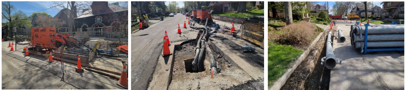
Figure 3 - Underground Sewer By-Pass System
