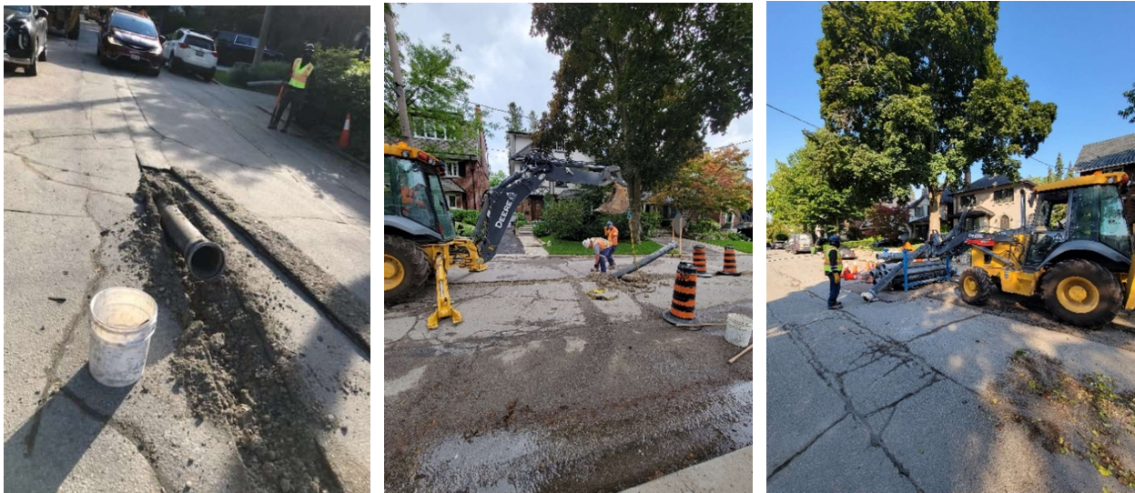
Figure 6 - Removal of the Underground Sewer By-Pass System
