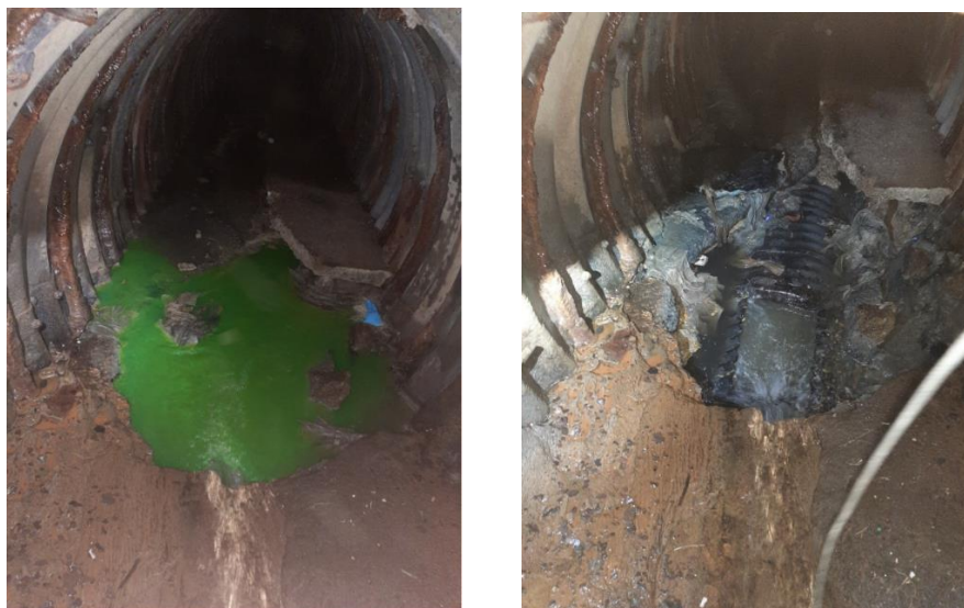
Figure 2: Photos of the failed sanitary sewer encased in concrete
