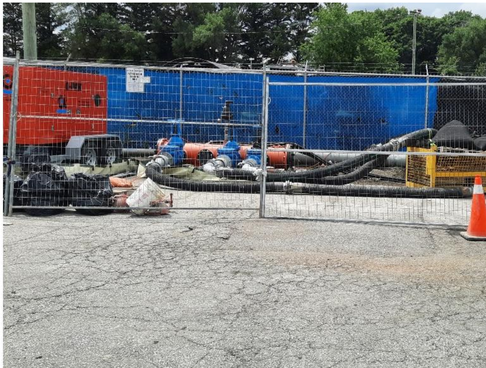
Figure 3: Storm & Sanitary bypasses
