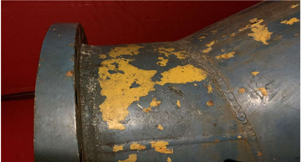
Figure 9 - Existing Coating on Exterior of Elbow
