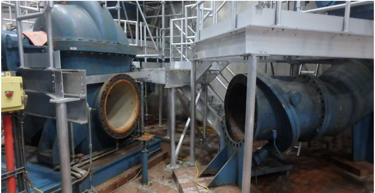
Figure 3 - Raw Water Pipes Demolishing
