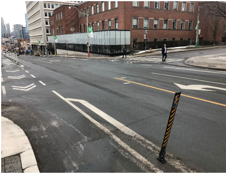
Figure 2: A new left-turn lane was installed on Yonge Street at Jackes Avenue-Farnham Avenue
