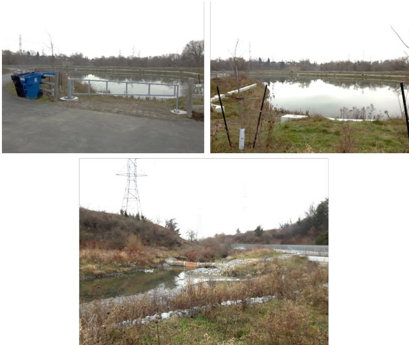
Figure 3: Top left image of Emery Creek Pond looking west. Top right image Emery Creek looking east. Bottom image of Emery Creek diversion weir.
