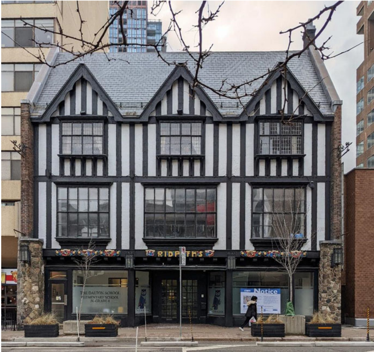
View of the east (principal) elevation of 906 Yonge Street (Heritage Planning, 2021)
