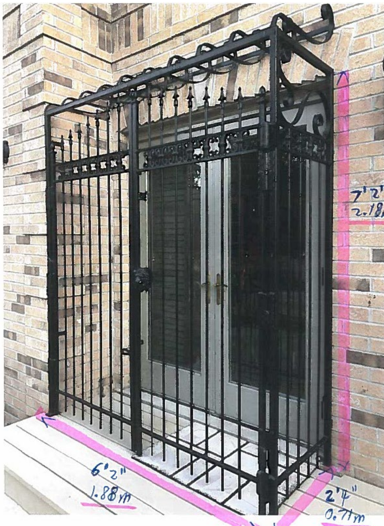
Attachment 3: Rear of house – basement egress east side
