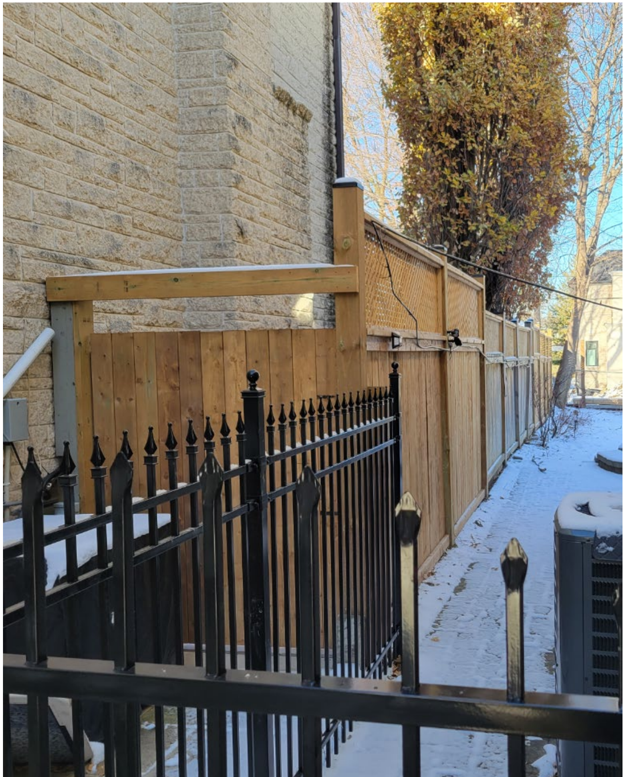
Attachment 2: Photo of fence – 54 YORK RD
