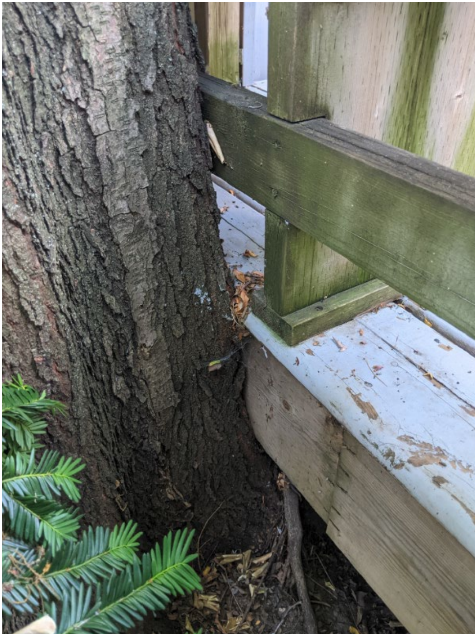
Attachment 2 – Figure 2: Arborist Report photograph showing the honey locust tree at the rear of 295 Woburn Avenue contacting the attached wooden deck
