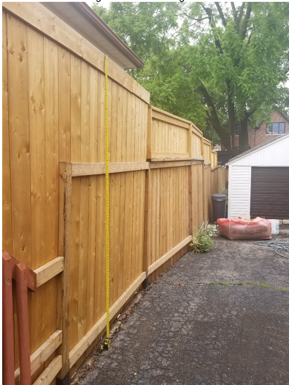
Attachment 2- Flankage Yard - 631 Glengrove ave- closer view of subject fence
