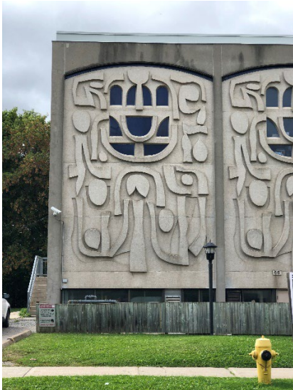
(Top) View of 55 Yeomans Road from northwest showing entrance. Heritage Planning, 2023. (Lower Left) View of prefabricated concrete bas-relief panels with stained-glass openings. Heritage Planning, 2023. (Lower Right) Map of the area showing 55 Yeomans Road in blue. Note: This location map is for information purposes only; the exact boundaries of the property are not shown. City of Toronto Mapping.
