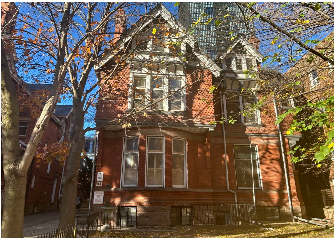
Figure 10: South elevation of 94 Isabella Street (Heritage Planning 2022).
