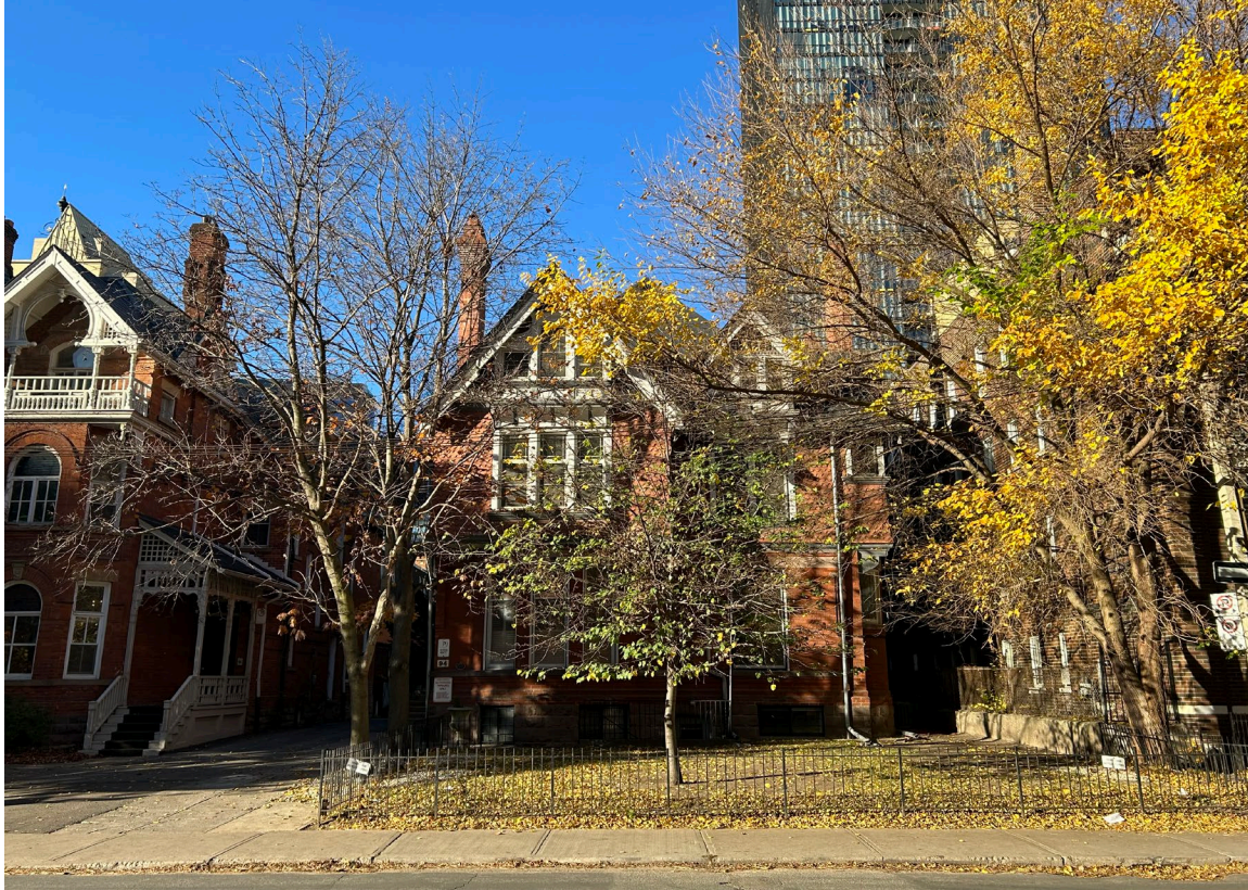
Figure 9: South elevation of 94 Isabella Street in context; 92 Isabella Street visible at left (Heritage Planning, 2022).
