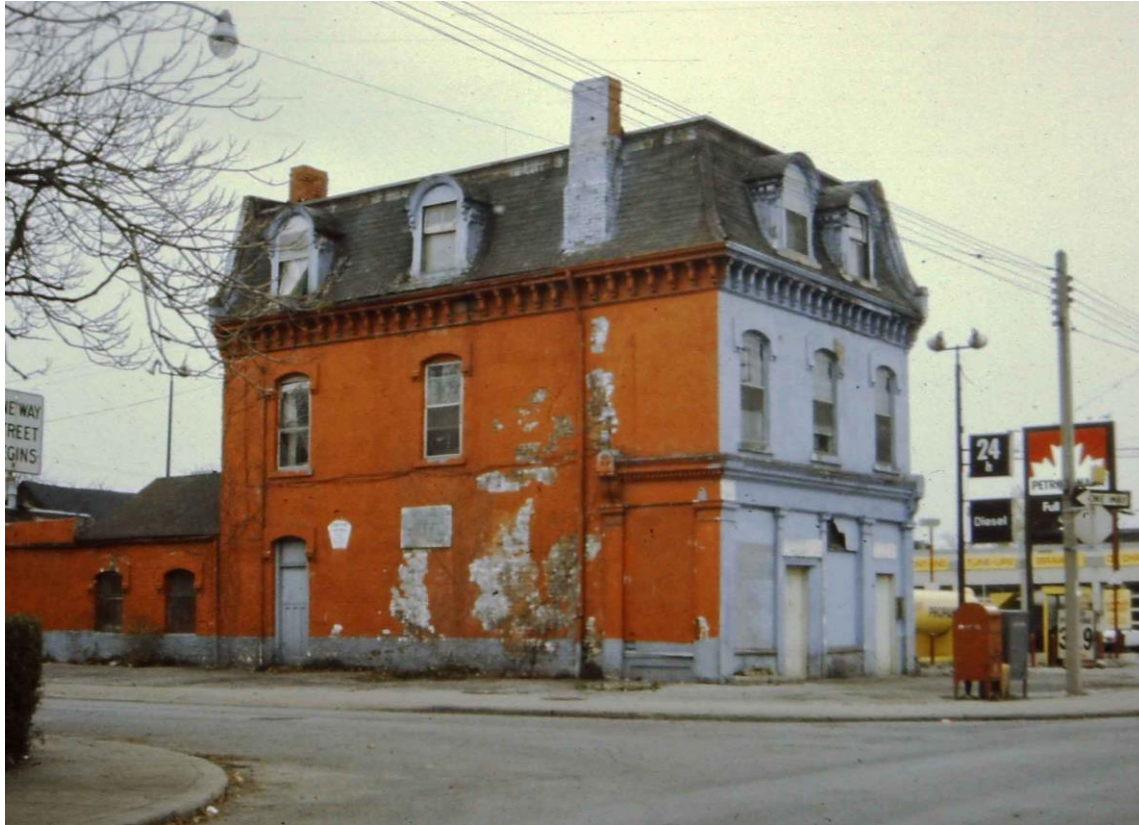
Archival photograph c.1991 (Toronto Historical Board, City of Toronto Archives)
