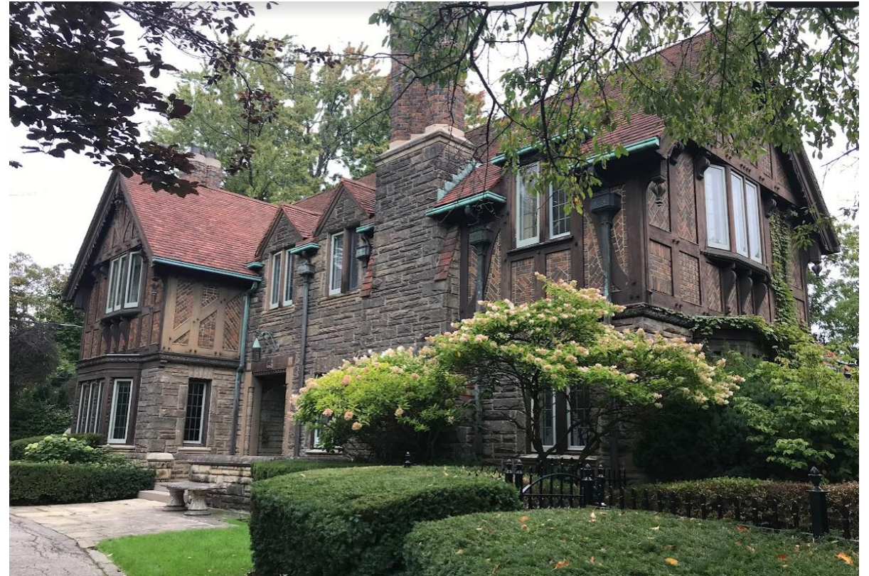
The west and partial south elevations of the subject property
