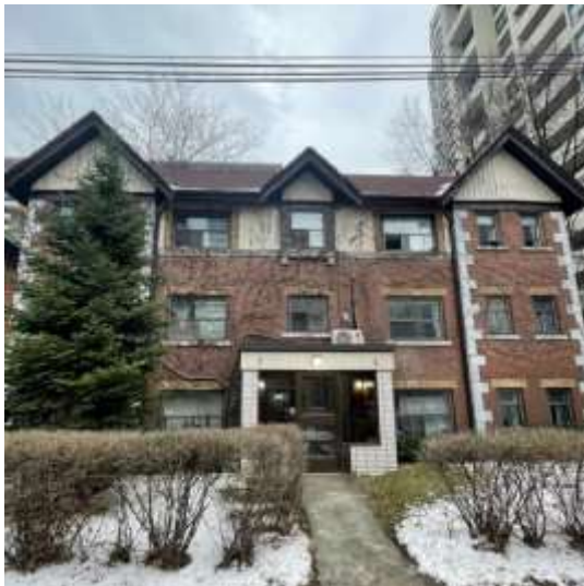
33 Maitland Street, Heritage Planning 2022.
