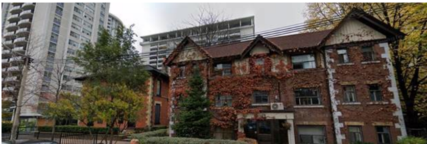
33 Maitland Street (R) in context with 37 Maitland St (L), Heritage Planning, 2022
