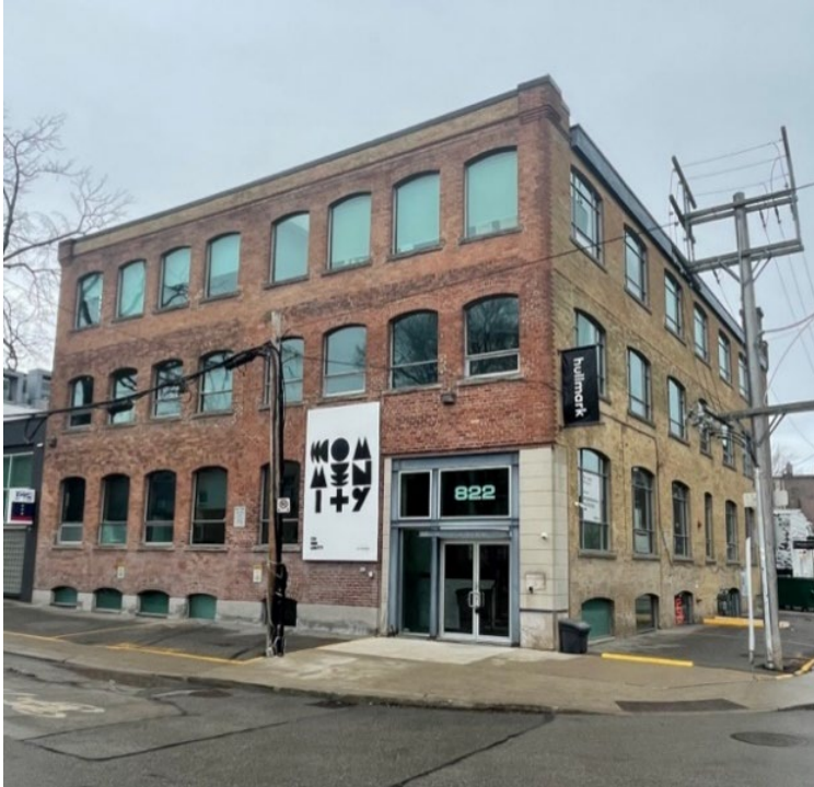
822 Richmond Street West, south façade, Heritage Planning, 2022
