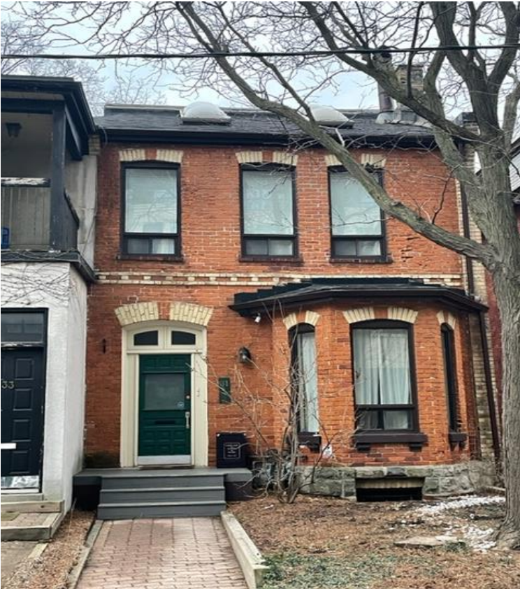
31 Linden Street, north façade, Heritage Planning, 2022
