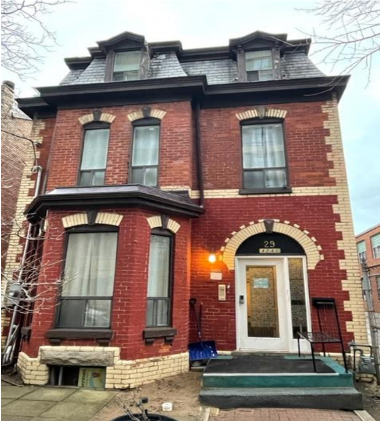
29 Linden Street, north façade, Heritage Planning , 2022
