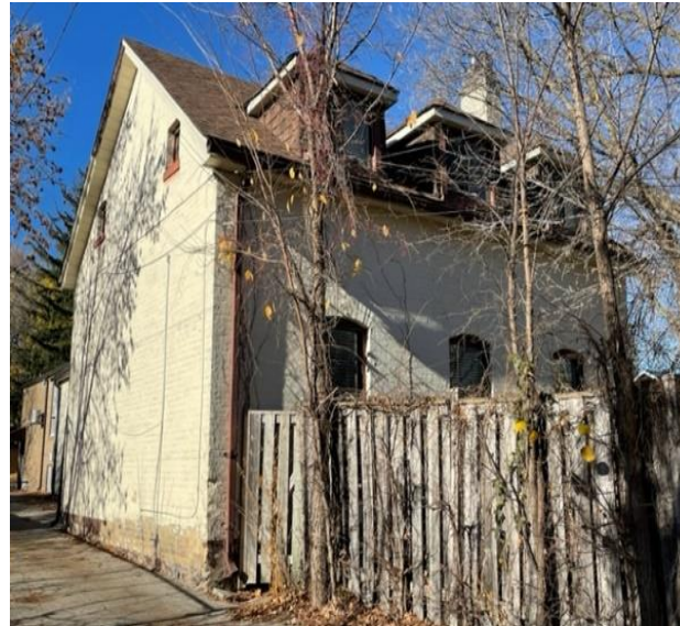
33 Melrose Avenue, Residence east façade, Heritage Planning, 2022
