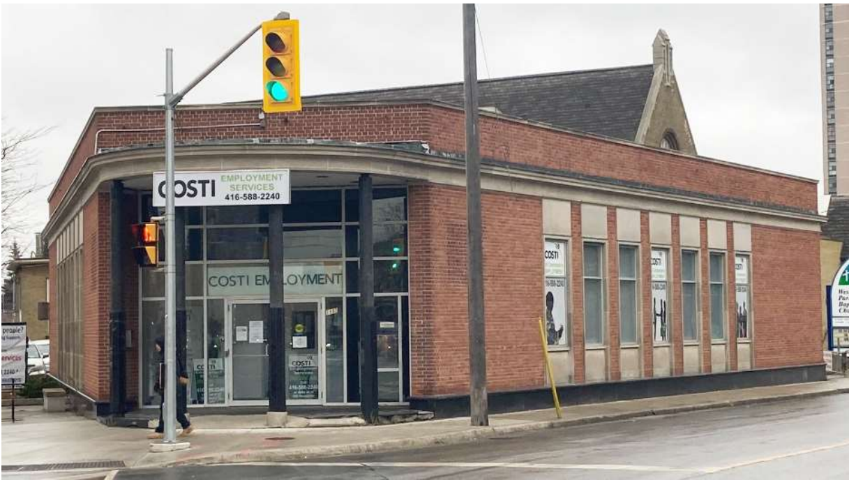
1885 Weston Road, Heritage Planning, 2023
