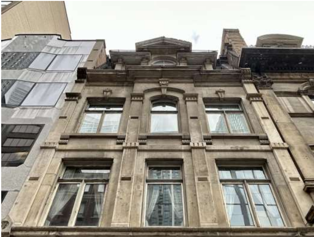
Figure 14: Limestone-clad upper storeys of 51 Yonge Street, 2023 (Heritage Planning).
