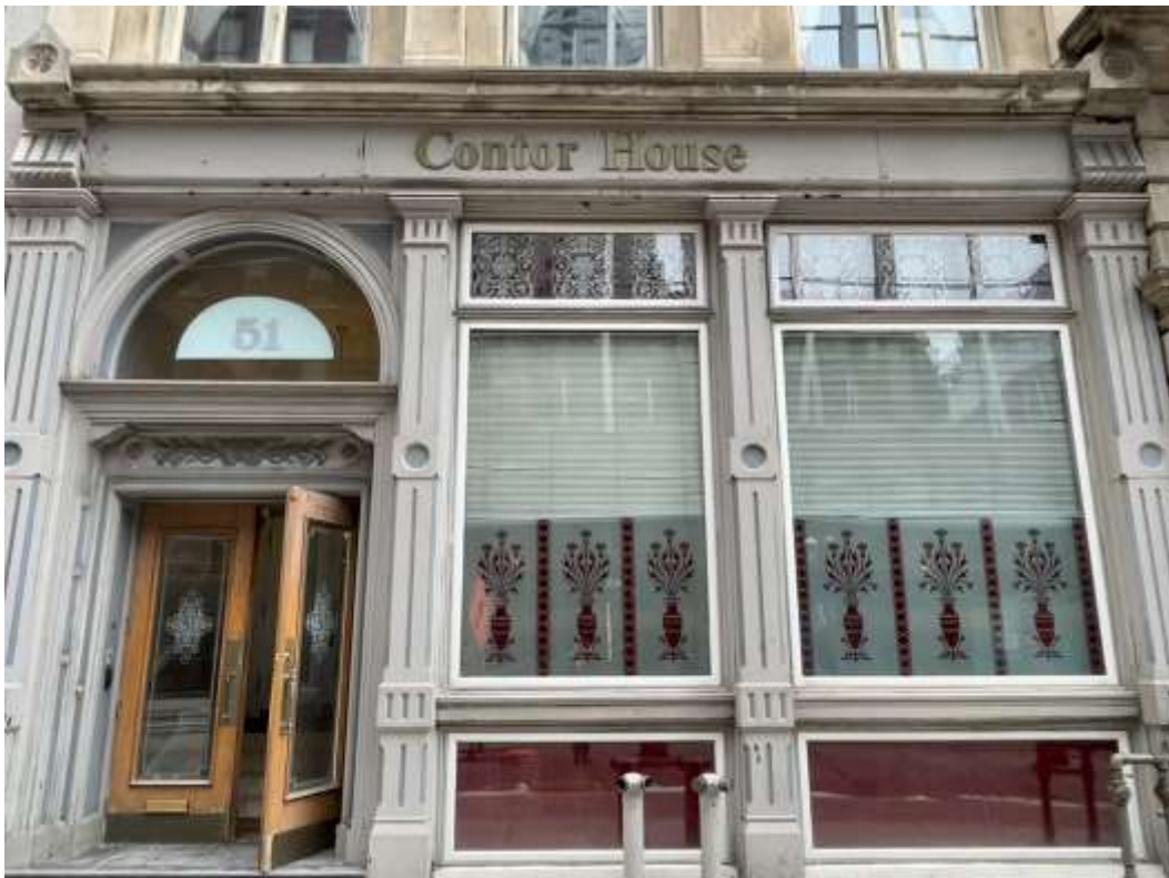
Figure 13: Ground storey storefront of 51 Yonge Street, 2023 (Heritage Planning).
