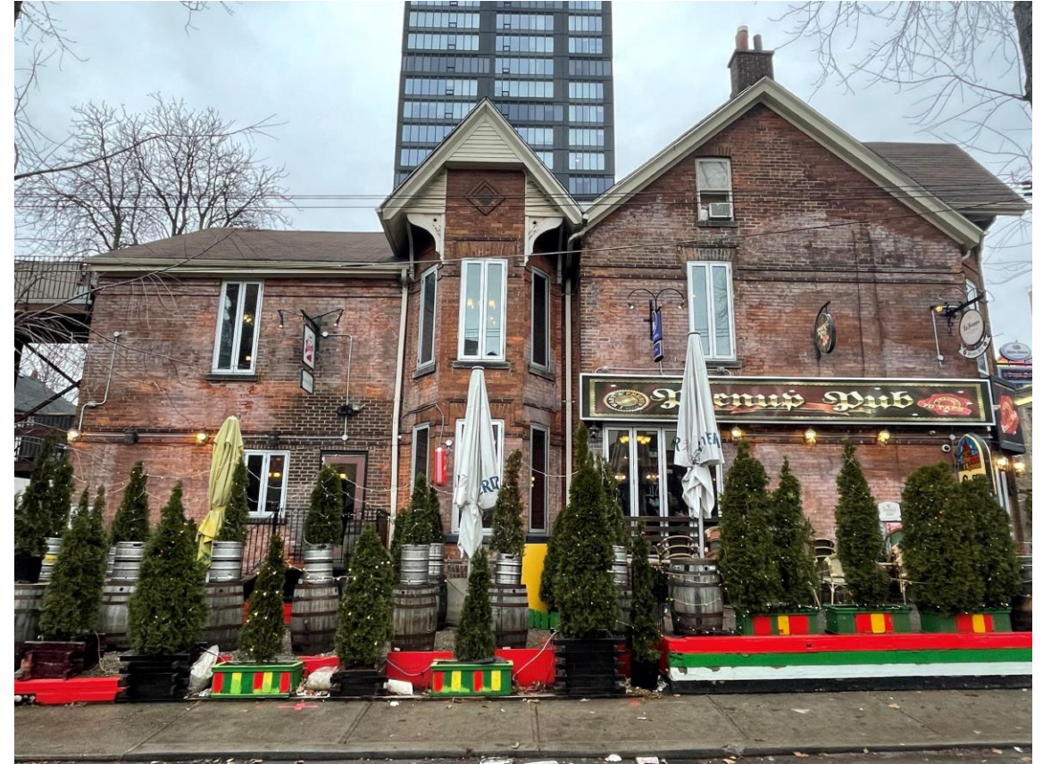
191 College Street – East elevation (Heritage Planning, 2022)
