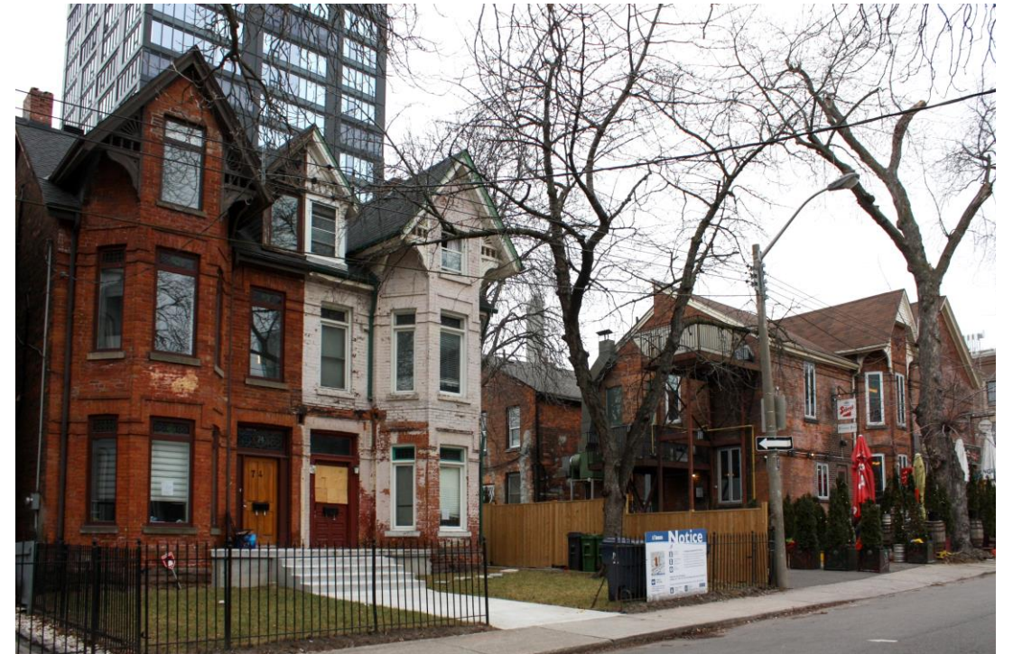
74-76 Henry Street (191 College Street visible at right) (Heritage Planning, 2023)
