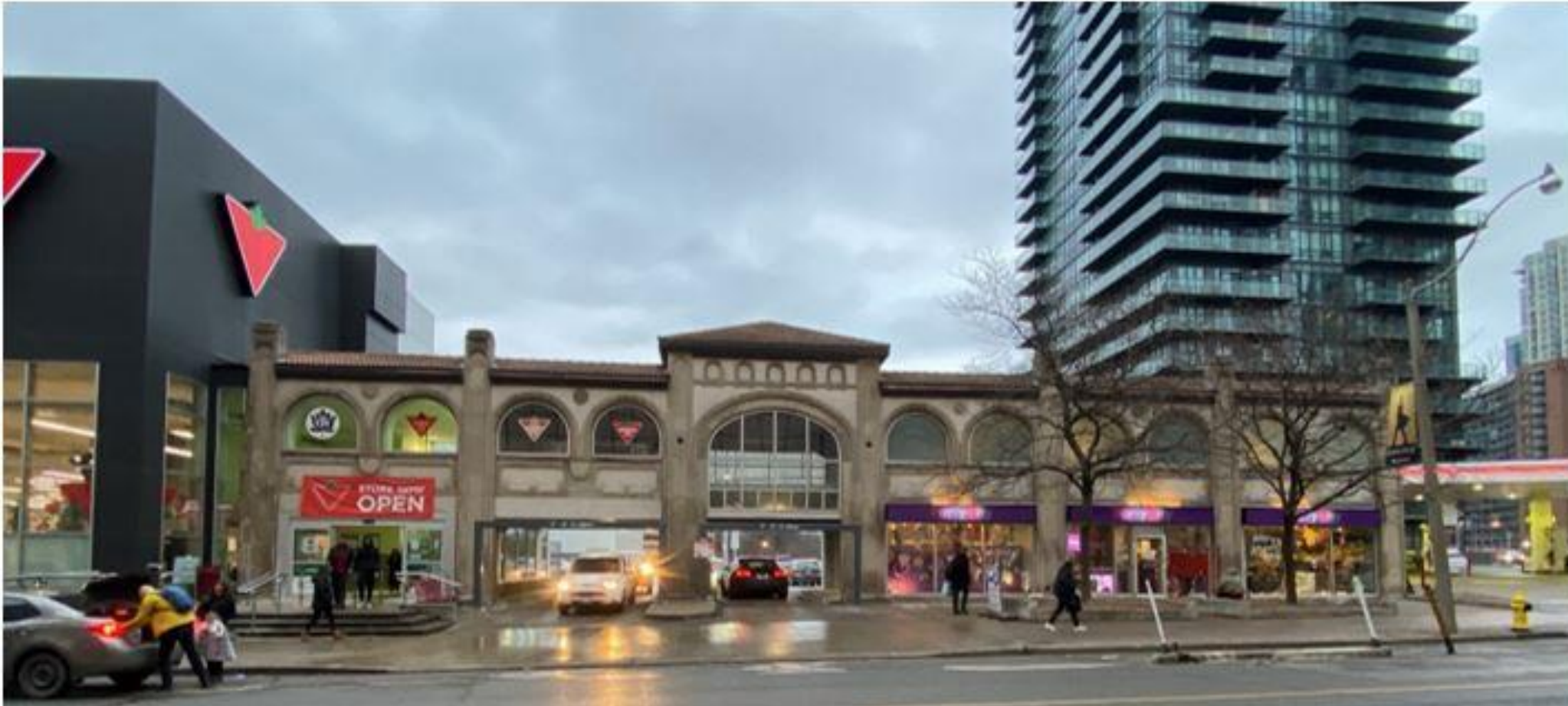
835 and 839 Yonge Street, west elevation of the Grand Central Market building (Heritage Planning, 2022)
