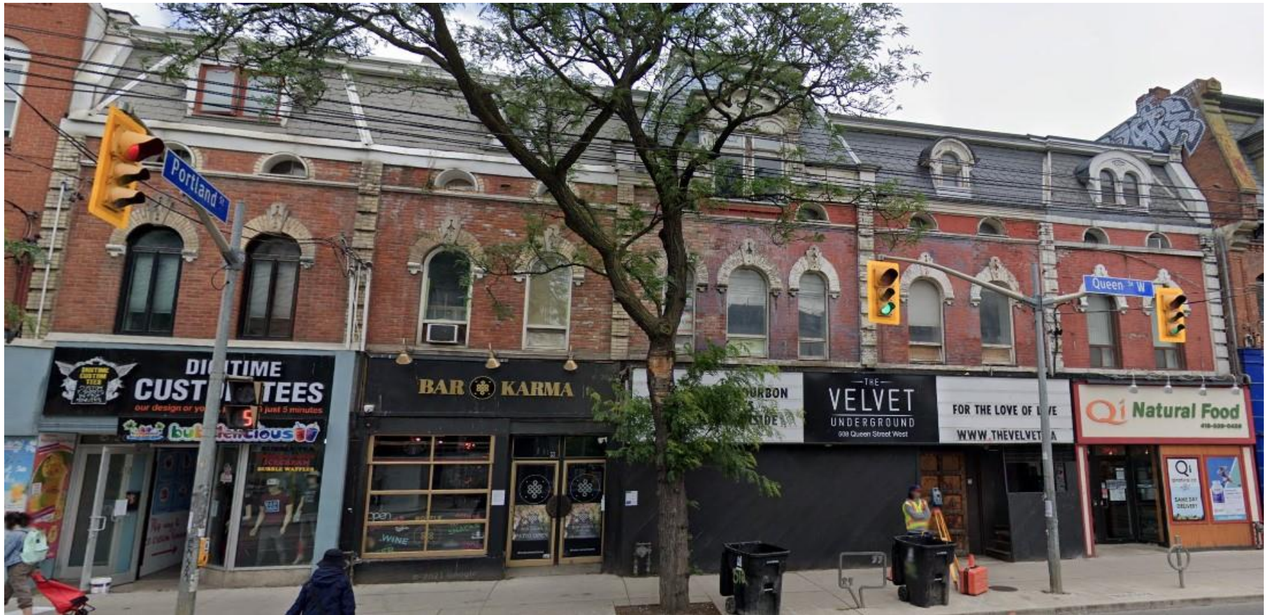
506-514 Queen Street West - designed by William Stewart in 1874; a contributing property of the Queen Street West Heritage Conservation District (photo source: Google)
