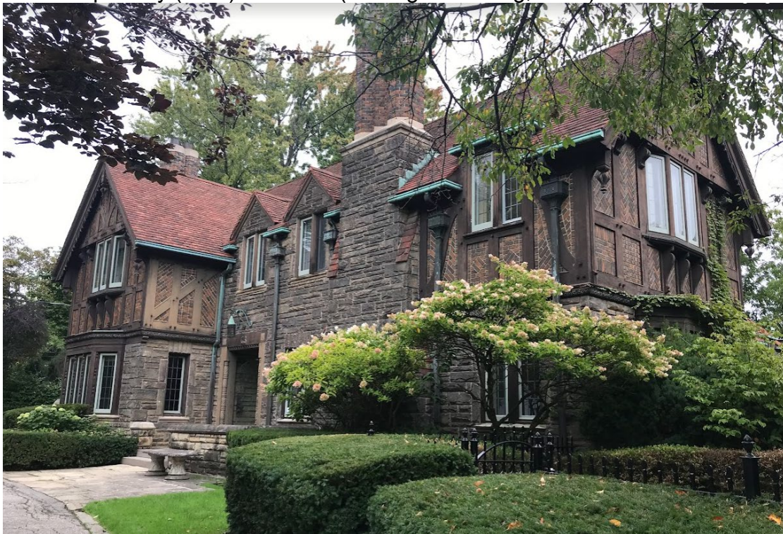
Photo of primary (west) elevation and partial south elevation (Heritage Planning, 2022)
