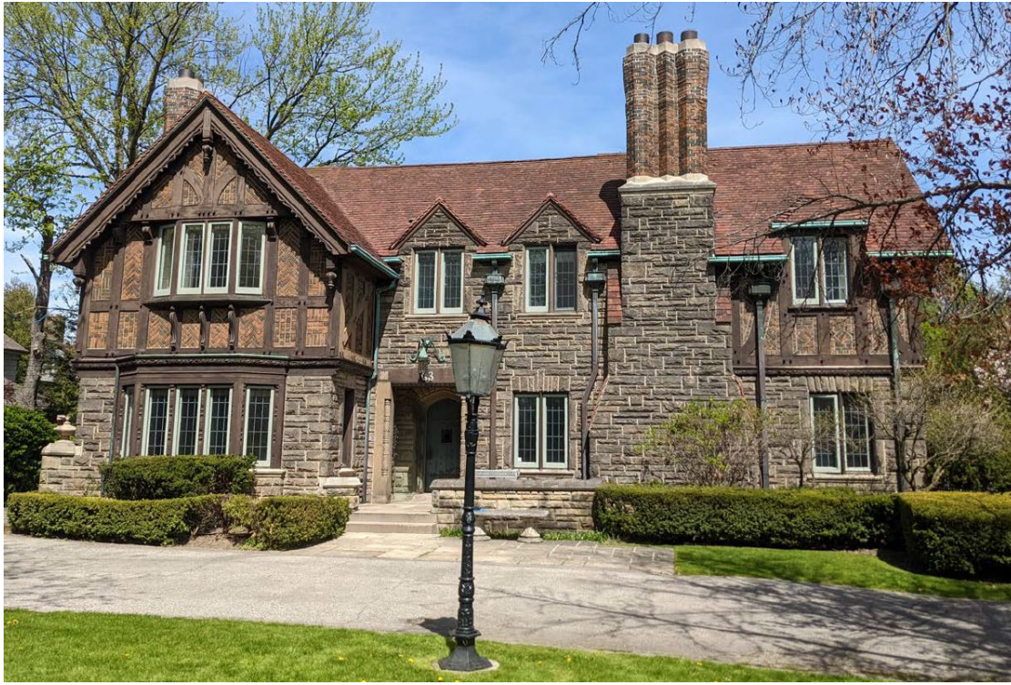
Photo of primary (west) elevation (Heritage Planning, 2022)
