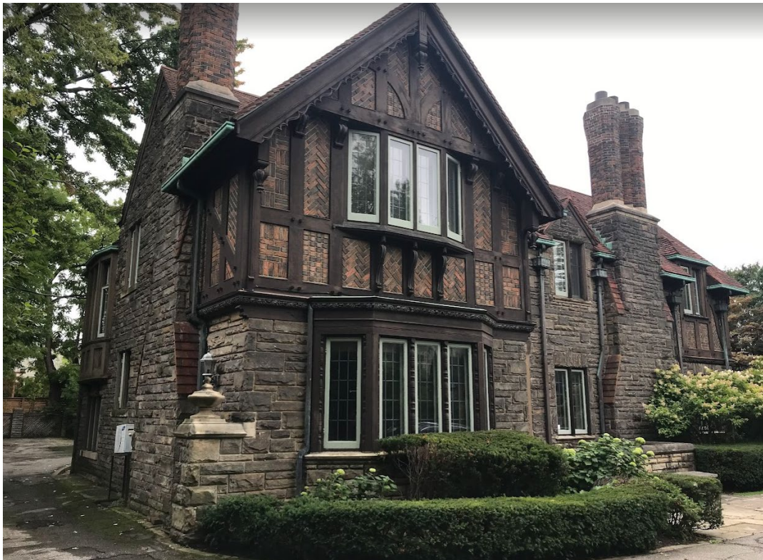
Photo of west elevation and partial north elevation (Heritage Planning, 2022)
