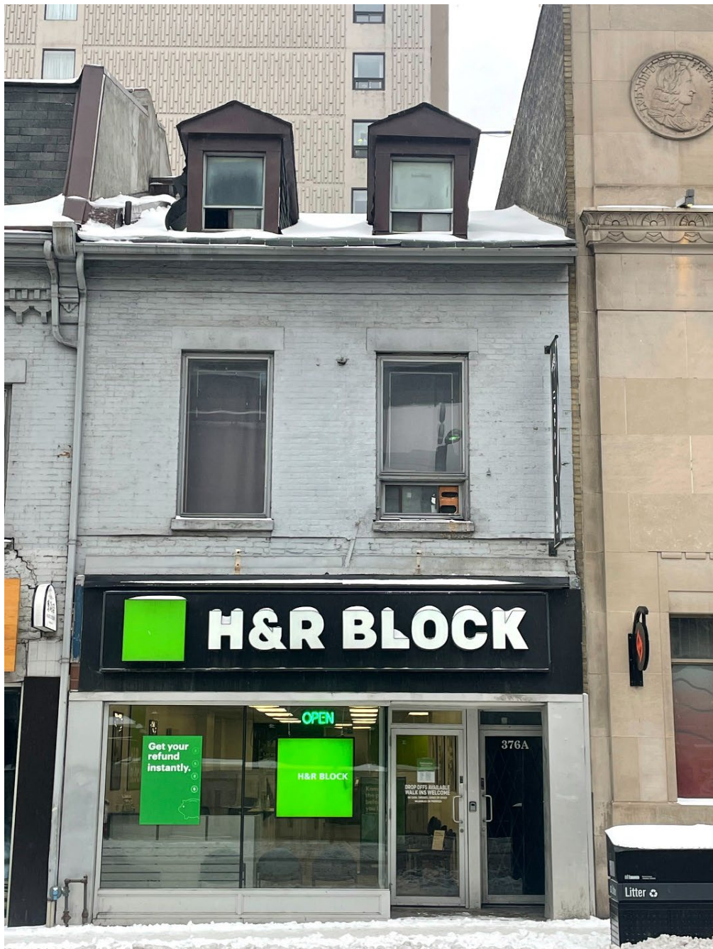
Figure 10: East elevation of 376 Yonge Street, 2023 (Heritage Planning)
