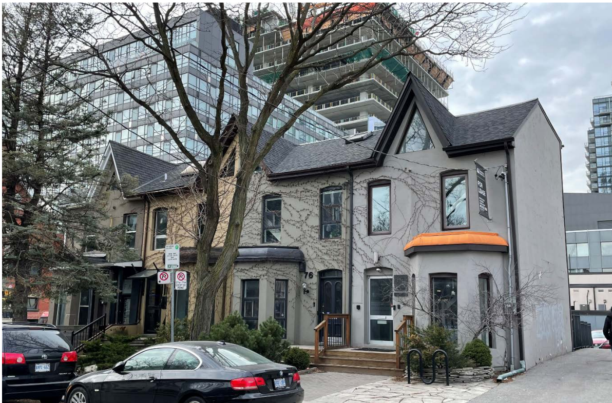
Current photo of the east elevations of the properties at 72-78 Berkeley Street. (Heritage Planning, Dec 2022)
