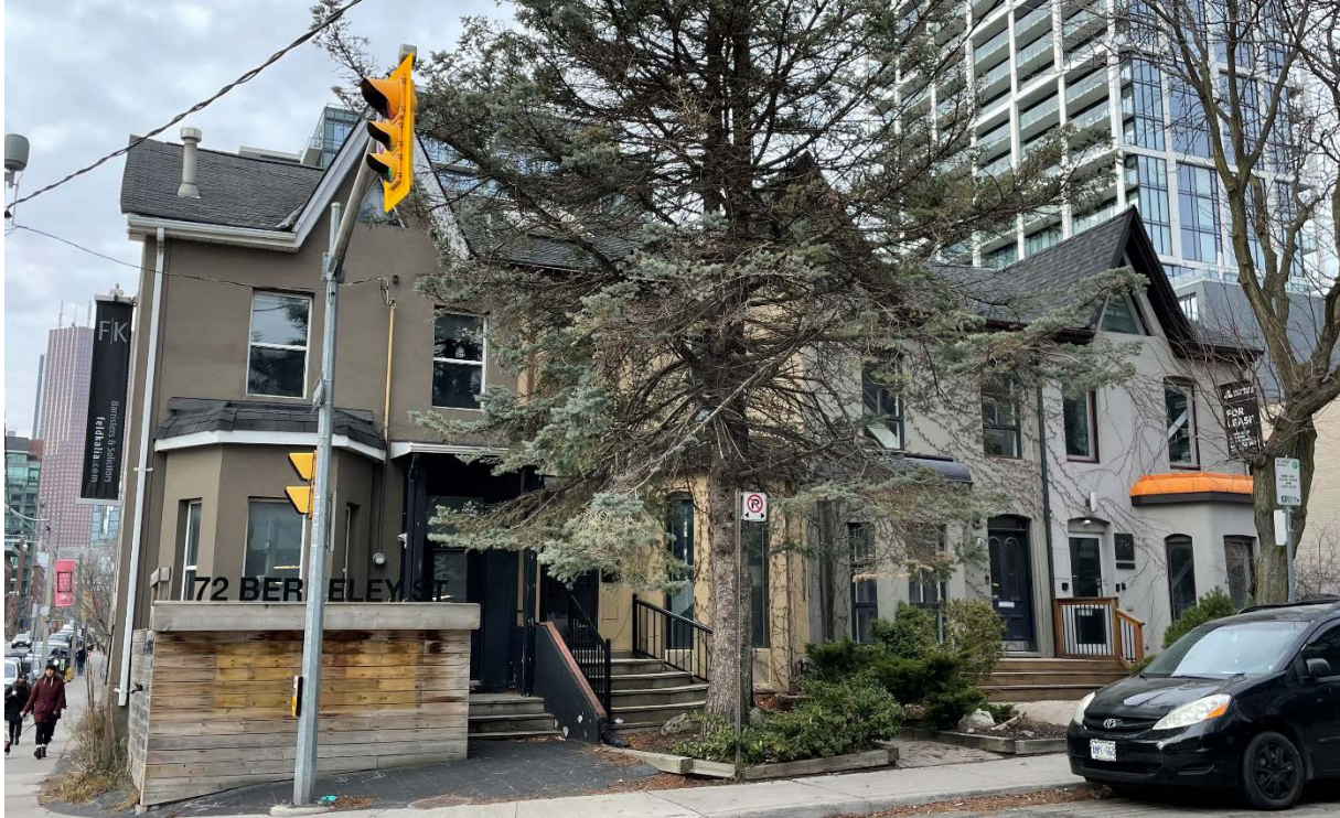
Current photo of the east elevations of the properties at 72-78 Berkeley Street. (Heritage Planning, Dec 2022)
