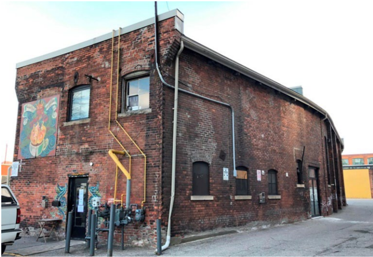
North and west facades of the powerhouse building showing the angled wall which was altered to accommodate the railway spur (HP, 2020)
