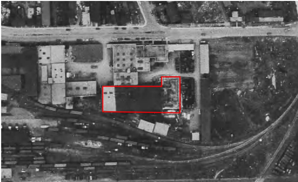
Figure 23: 1947 Aerial photograph, showing the completed western addition (distinguishable by variation in roof colour), and the eastern addition, which appears to be under construction at the time the image was captured. The red outline indicates the completed building perimeter of 185 Eastern Avenue. (City of Toronto Archives, annotated by Heritage Planning)
