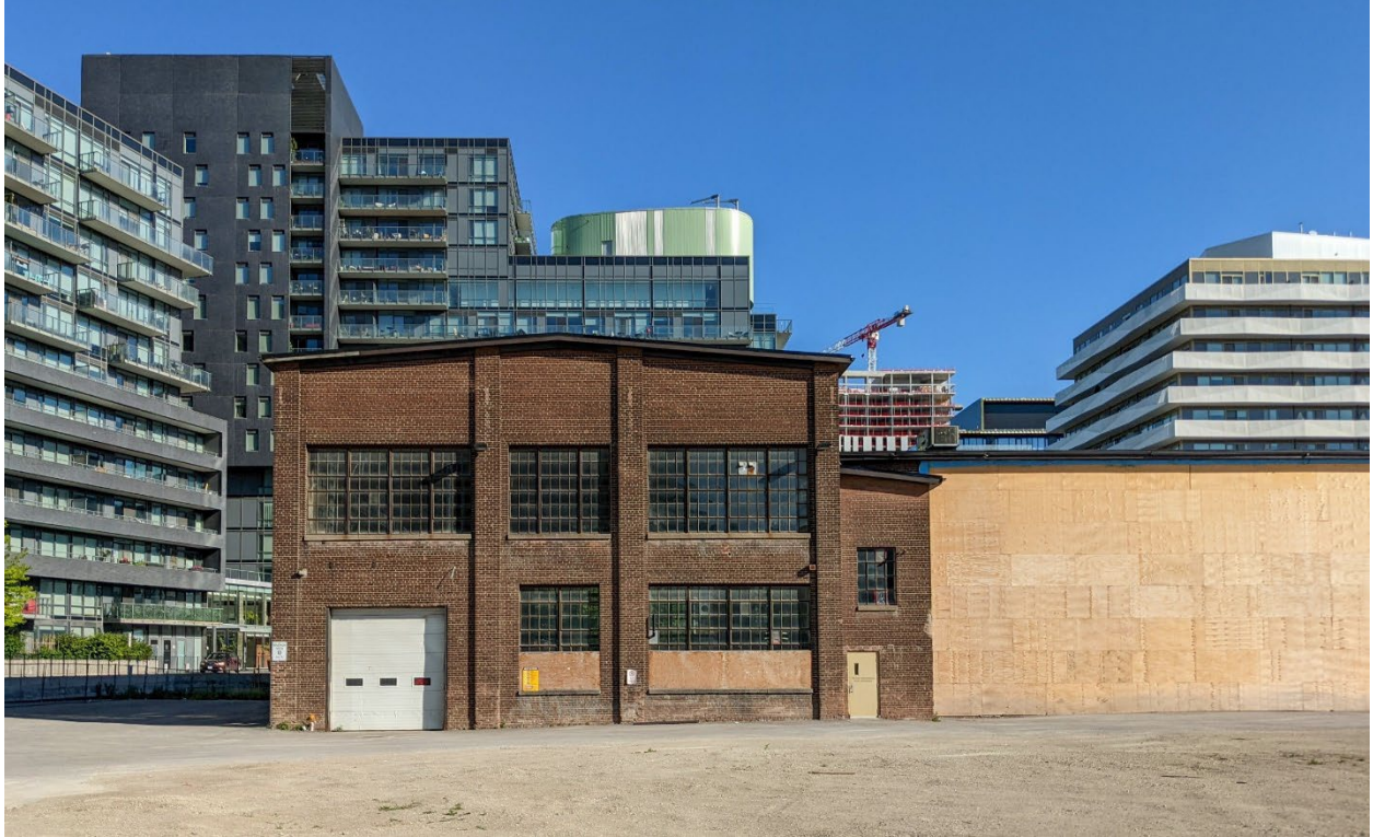
Figure 28: Partial north elevation of 185 Eastern Avenue. (Heritage Planning, 2022)
