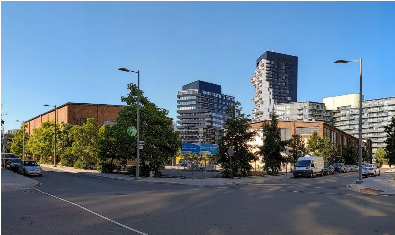
View of 153 Eastern Avenue and 185 Eastern Avenue from the southwest (Heritage Planning, 2022)
