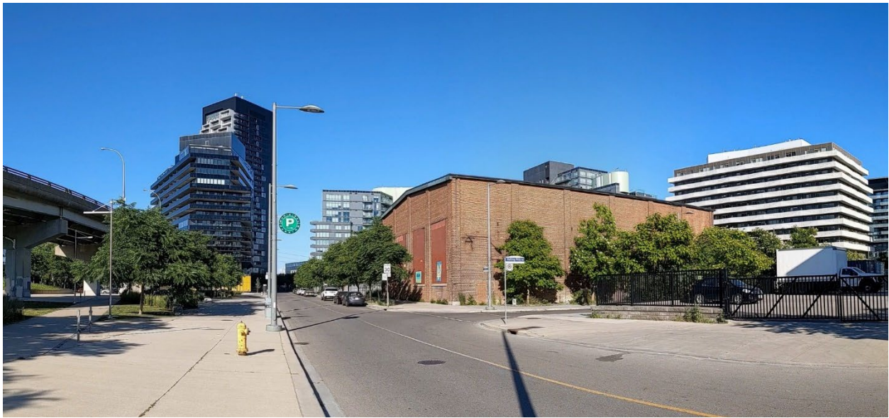
Figure 41: View east on Eastern Avenue, showing the Cleaning Room (153 Eastern Avenue) anchoring the site at the corner of Rolling Mills Road and Eastern Avenue. The major infrastructure intervention for the Don Valley Parkway is visible north of the subject properties (on the left of the image), and recently constructed high-density residential projects surround the site to the east and south. (Heritage Planning, 2022)
