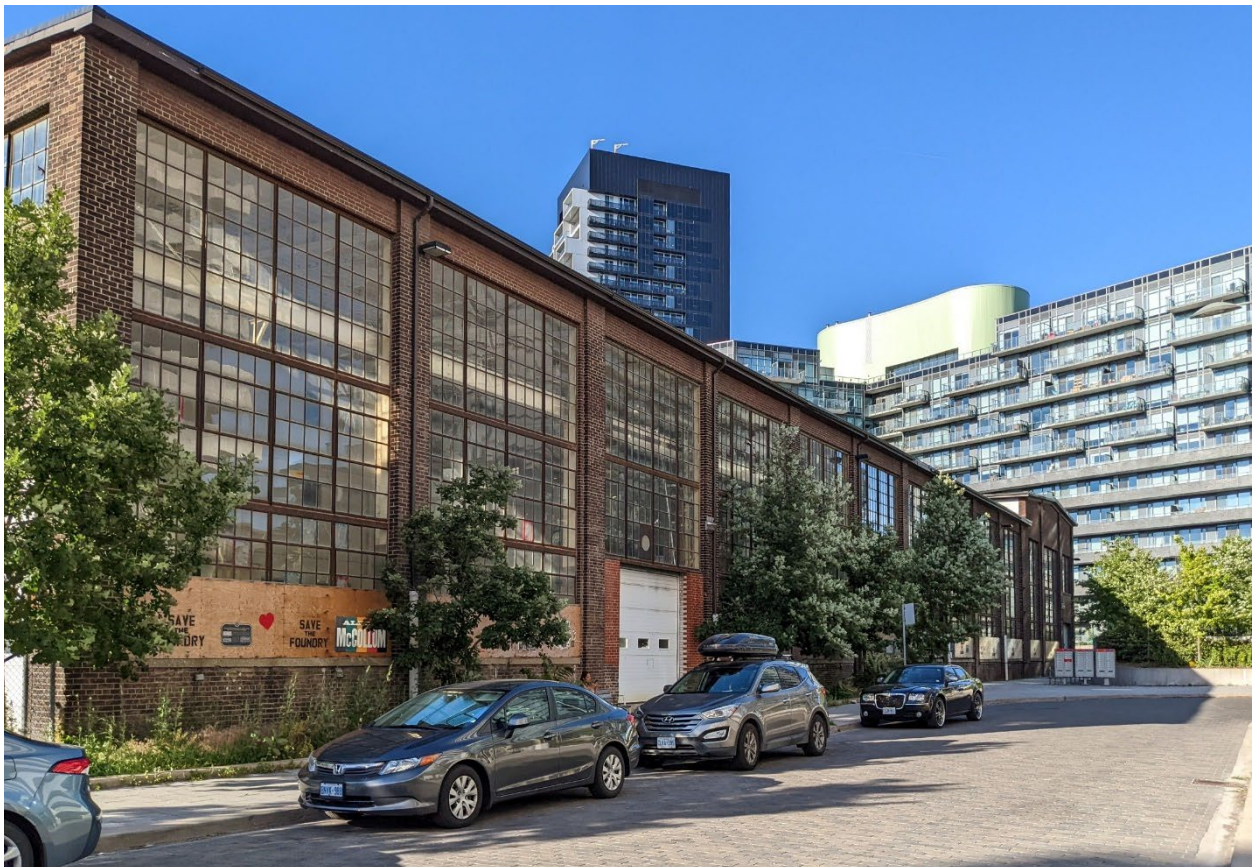
Figure 20: A reminder of the rail yards that no longer exist, 185 Eastern Avenue is oriented southward towards what is now Palace Street. The two bays in the foreground are the western addition from c.1946. (Heritage Planning, 2022)
