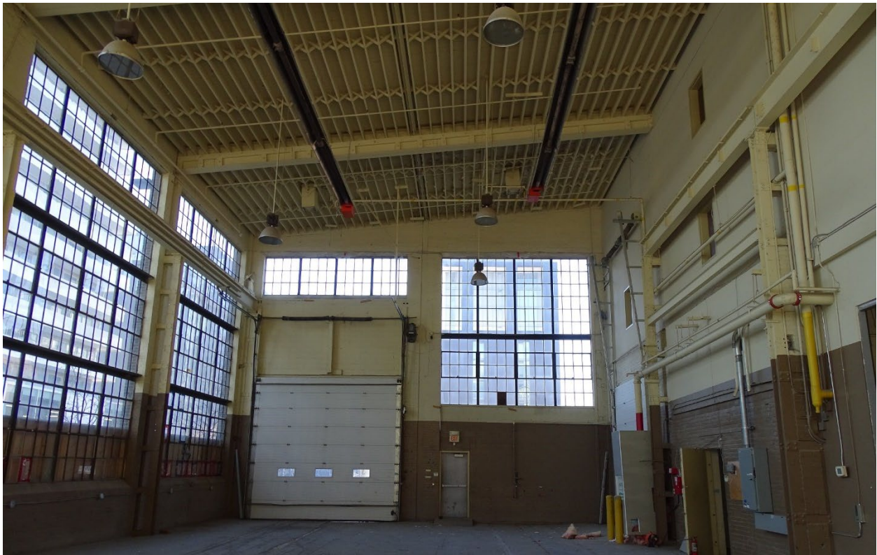
Figure 31: Interior photograph of 185 Eastern Avenue looking west, showing a closer detail of the roof structure in the western addition (SBA Ltd., 2021)
