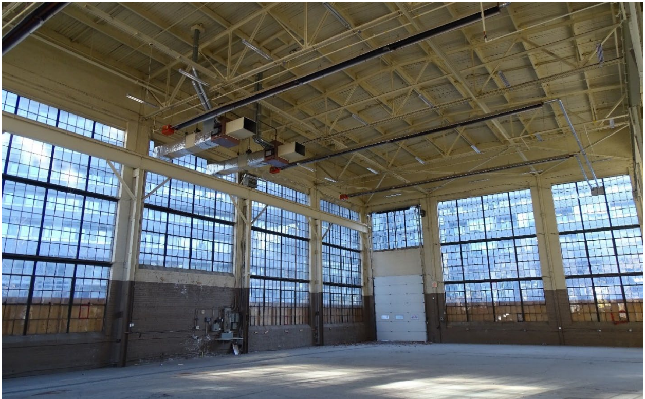
Figure 33: Interior photograph of 185 Eastern Avenue showing the eastern addition including steel roof trusses and gantry crane support structure, looking southeast (SBA Ltd., 2021)
