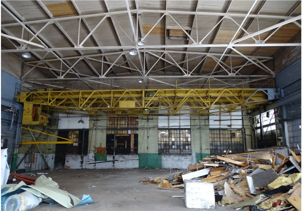
Figure 40: Interior photograph of 153 Eastern Avenue, showing the steel roof trusses, wood roof decking, and the steel gantry crane with secondary support structure. (SBA Ltd., 2021)
