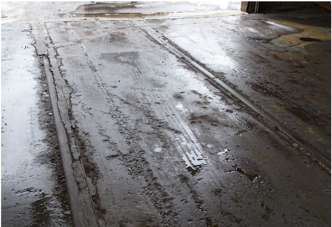
Figure 34: Interior photograph of 185 Eastern Avenue showing the detail of the railway tracks embedded in the concrete floor slab (SBA Ltd., 2021)
