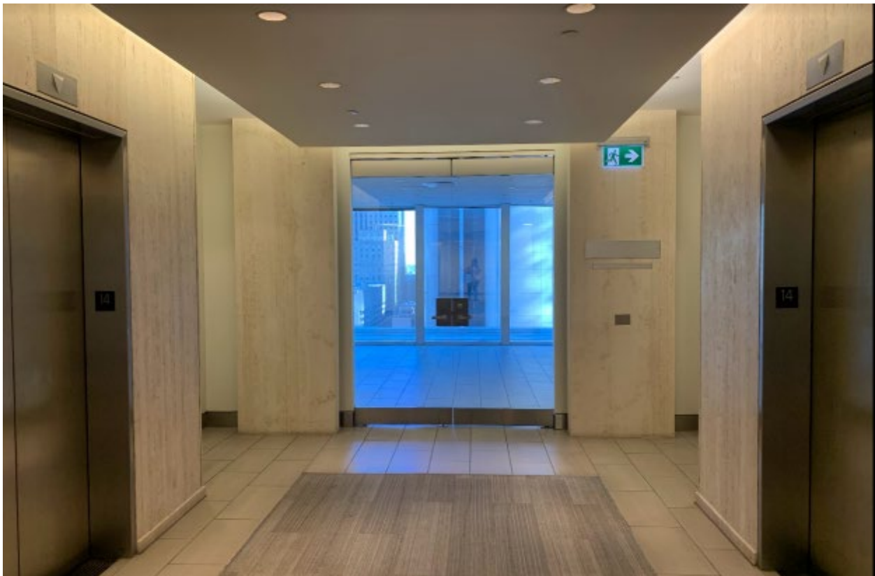
Image 45. Current photo on the fourteenth floor, looking east from the elevator lobby with its travertine wall panelling, stainless steel elevator doors and surrounds, and drop ceiling panel with recessed pot lighting (Heritage Planning, 2023)
