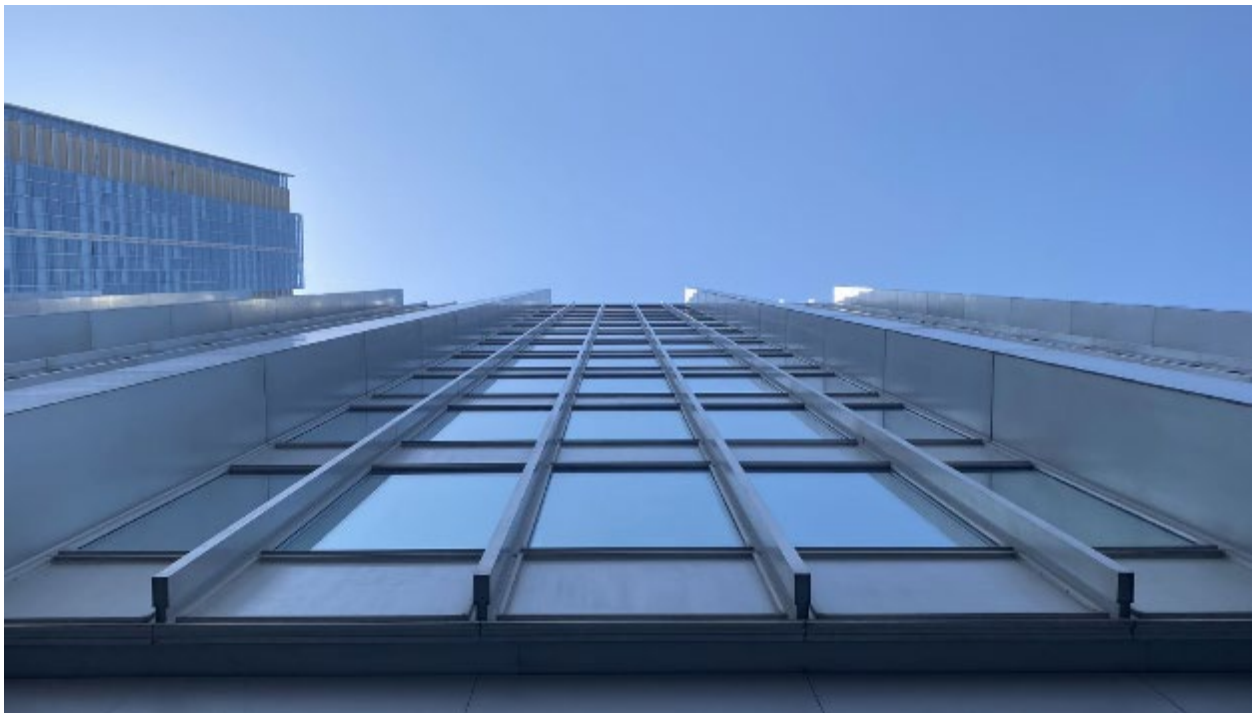
Image 37. Current photo looking up and showing the aluminum-clad "fins" (at centre) flanked by larger perimeter columns found on all four storeys of the building exterior and creating a strong sense of verticality. (ERA, 2022)
