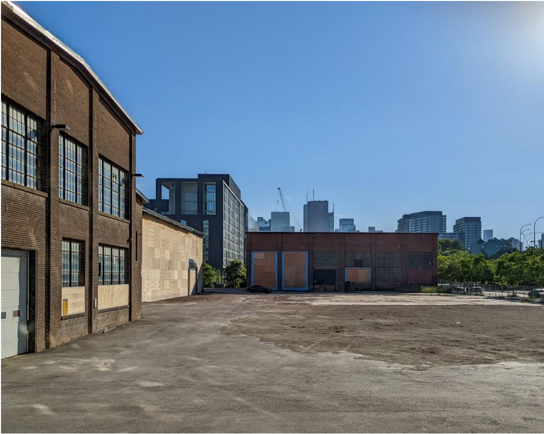
Current view of site, looking west towards 153 Eastern Avenue (Heritage Planning, 2022)
