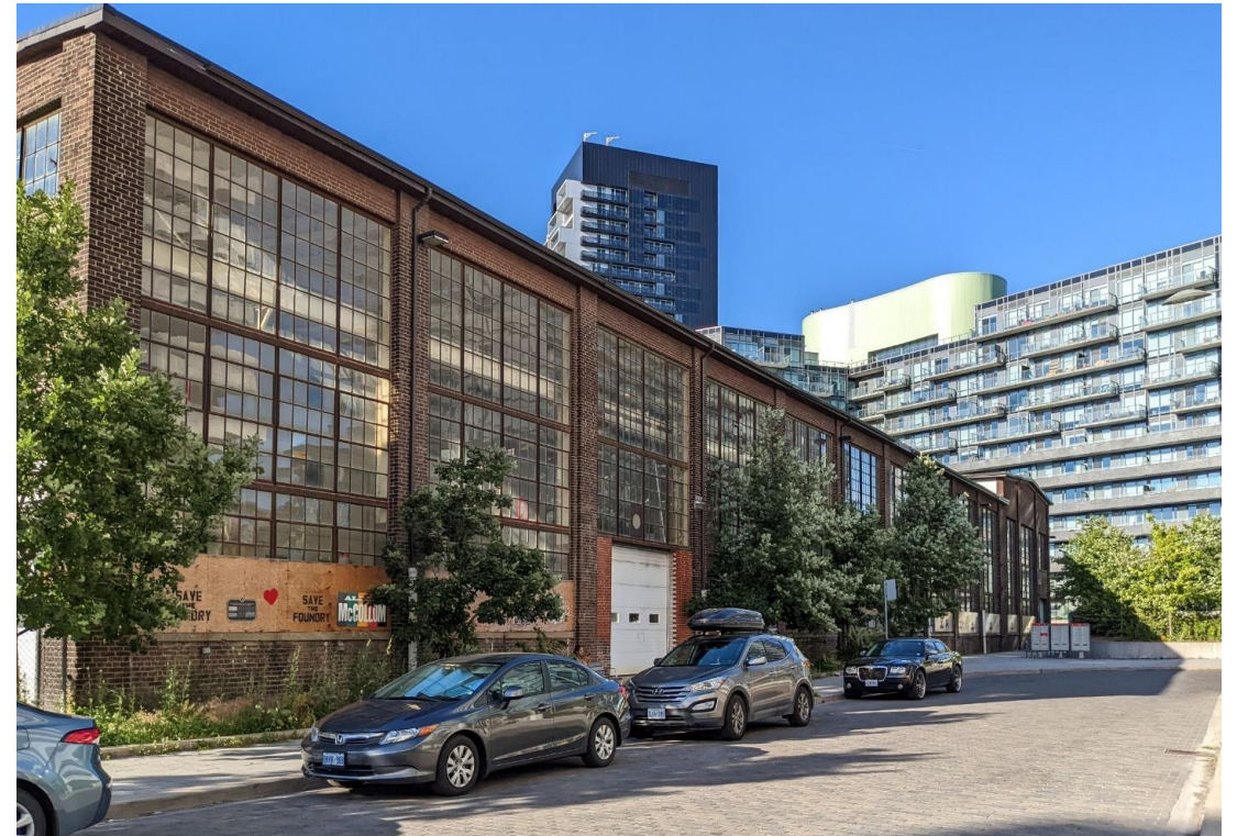
185 Eastern Avenue - south elevation (Heritage Planning, 2022)
