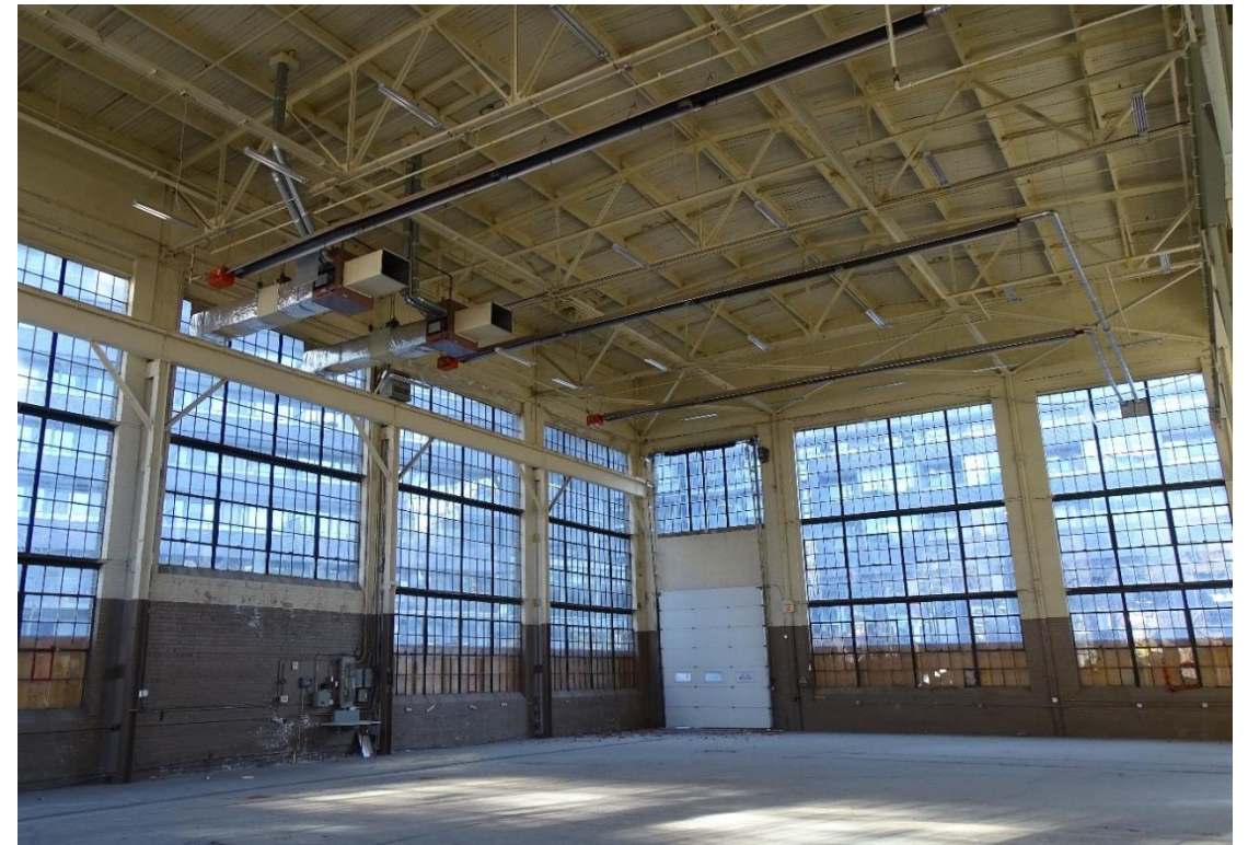
Interior of the Machine Shop, 185 Eastern Avenue (SBA Ltd., 2021)
