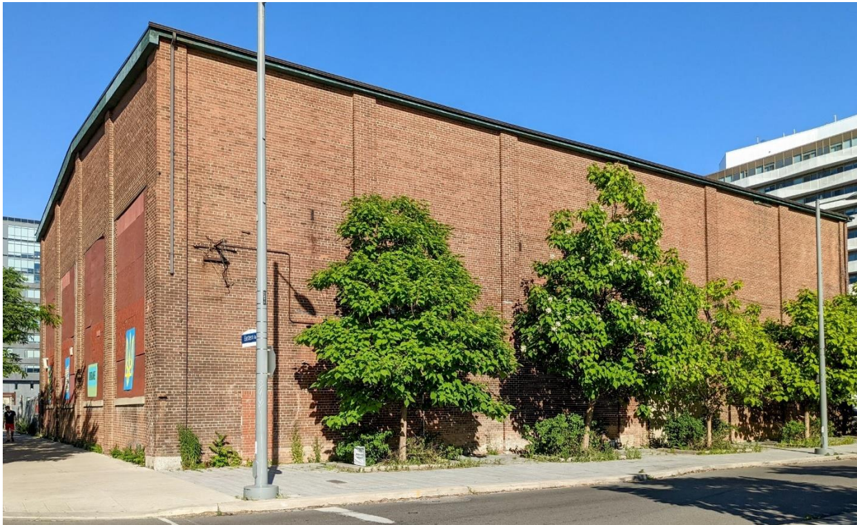
153 Eastern Avenue - north and west elevations (Heritage Planning, 2022)
