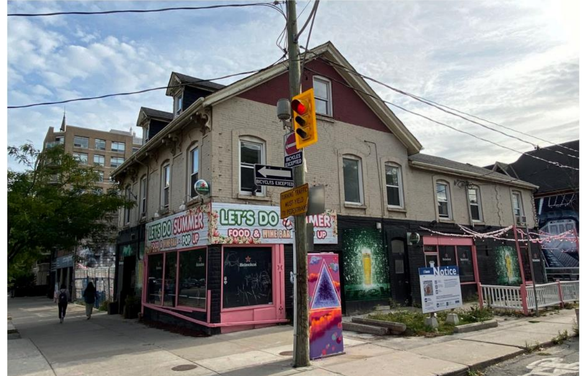
Existing North Elevation along Richmond St W
