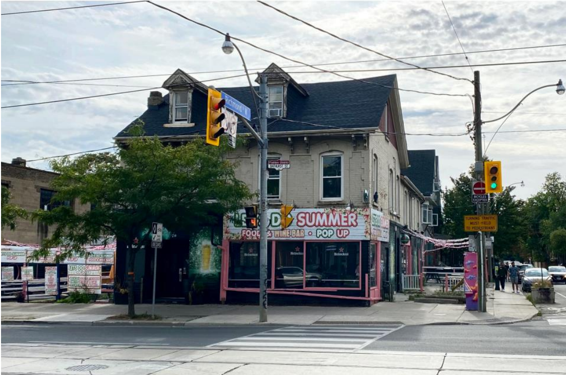
Existing East Elevation along Bathurst St
