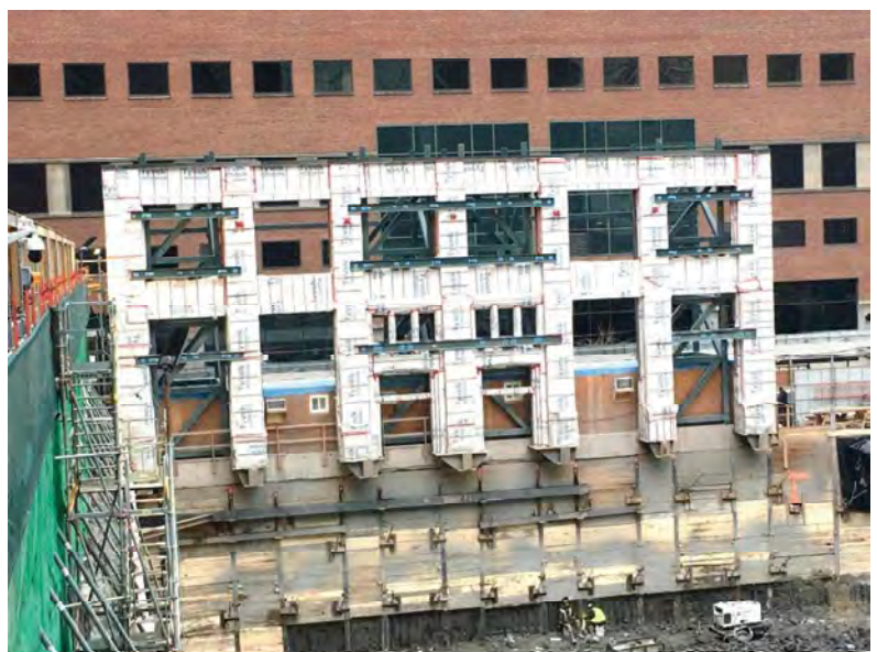
Cantilevered retention, interior needle beams
