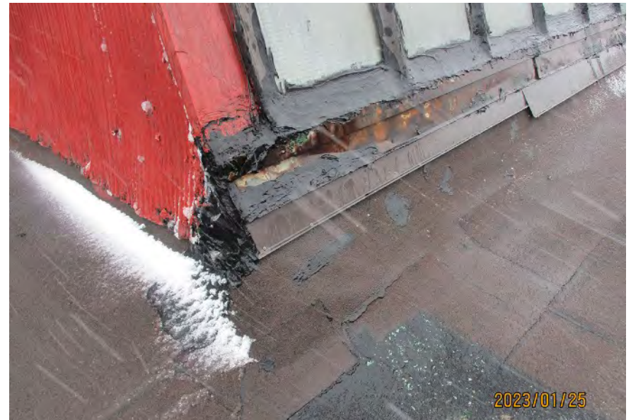
Close-up of a corner of a sawtooth skylight on the western portion of Building C. Note the heavy use of sealant throughout, which completely hides the steel frame profile. The bottom flashing is corroded and new flashing was added.
