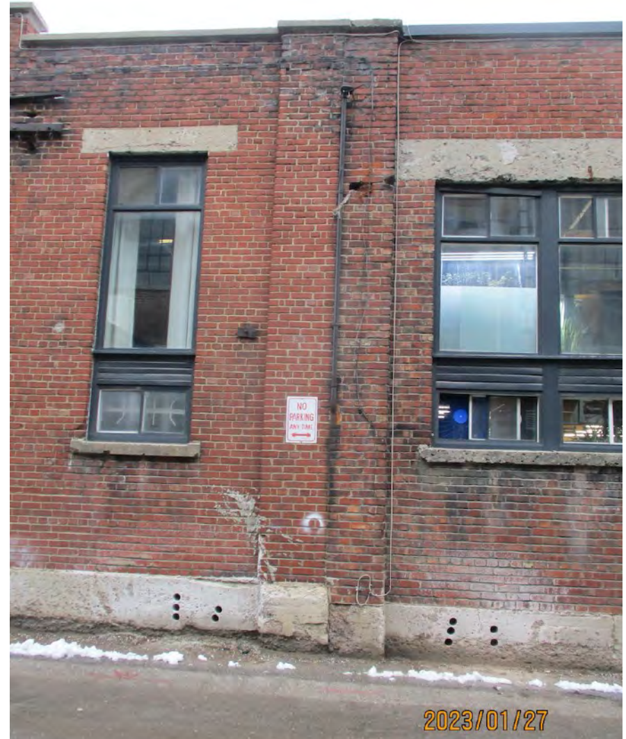
South elevation, at the junction between two construction periods (the western portion was built prior to the eastern portion) showing severely weathered brick parapet, localized corrosion staining at concrete lintel, weathered and heavily deteriorated window sills and brick staining due to water runoff and a lack of proper flashings or drip edges. Windows are wood and aluminum replacements (likely 1990s).
