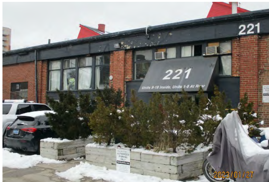
West elevation showing alterations to openings. Note the northern bay (left of the photo) was infilled with new bricks.
