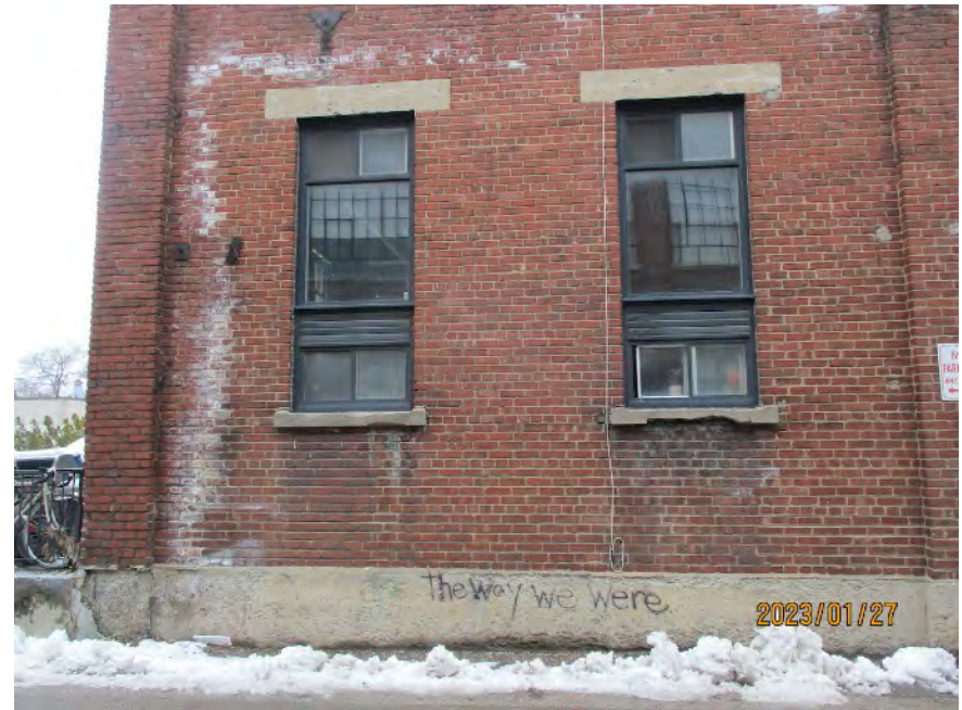
Building C (west) south elevation, showing weathered condition of brick wall, window sills and lintels, and concrete foundation. Of note is the heavy efflorescence near the corner. This efflorescence is also shown on the interior side, along with deteriorated masonry, likely due to faulty interior plumbing.
