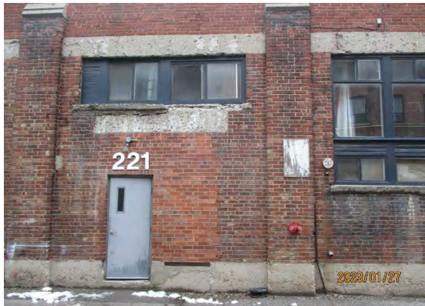
South elevation showing altered bay accommodating a smaller window and a door. Brick is heavily soiled below the cap stones above the pilasters and below window sills due to a lack of a proper drip edge below the cap stone.
