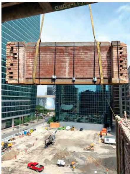
Spandrel with toothed pilaster
