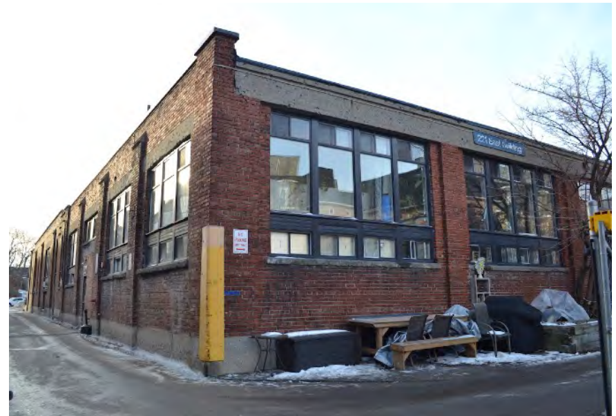
Corner of the south (left) and east(right) elevations. Window opening sizes and locations differ, as well as the wall compositions (on the east elevation, the concrete lintels are continuous along the length of the building, whether on the south elevation, lintels are interrupted). Sills on the east elevation are heavily eroded and do not project as much as the sills on the south elevation, resulting in more notable water run-off. In either case, the sills are lacking proper dip cuts/ grooves to break the flow of water.
