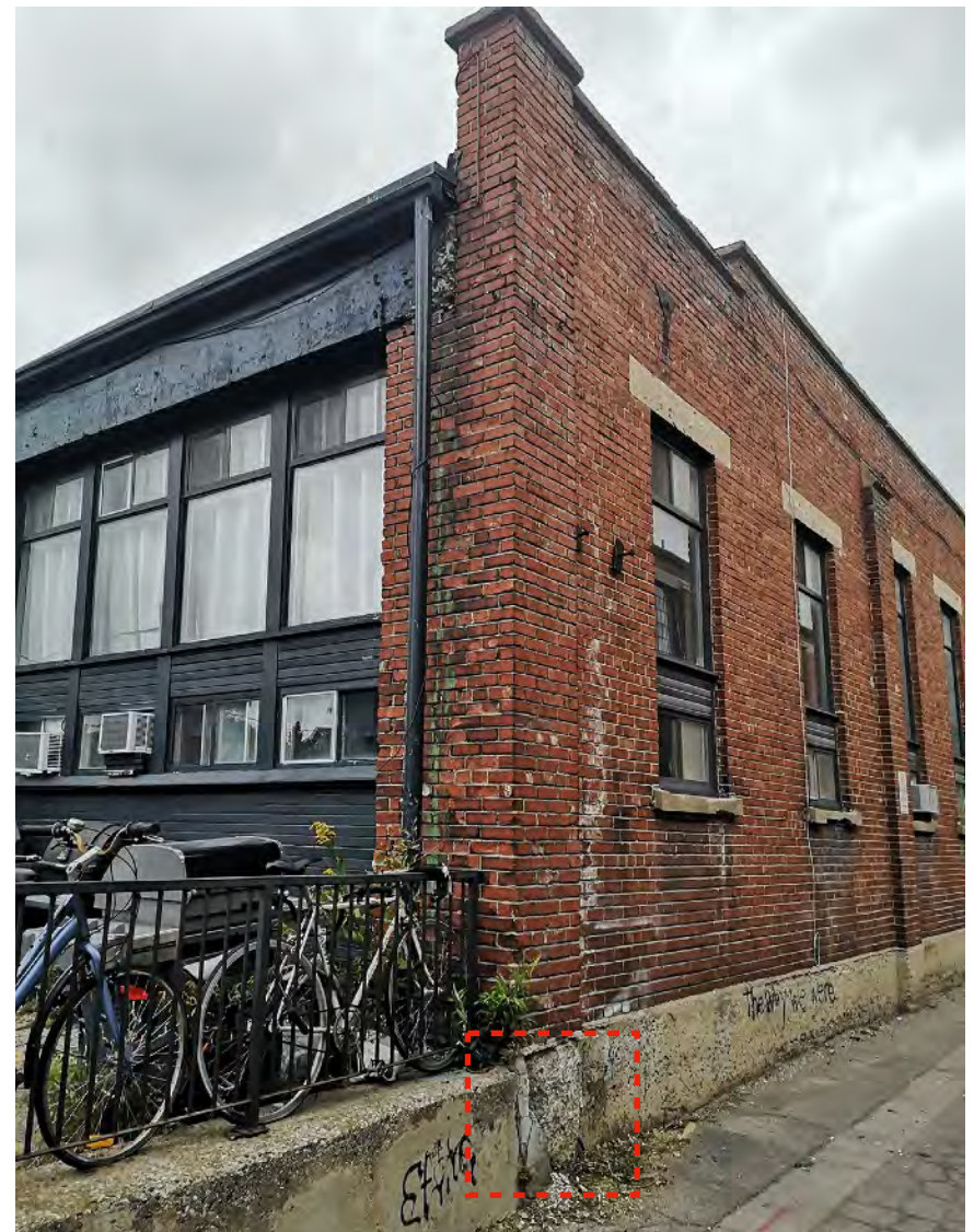
Corner of the west (left) and south(right) elevations. The edge of the concrete lintel of the west elevation is damaged. Also of note is the heavily spalled concrete base (close-up on the picture on the left).
