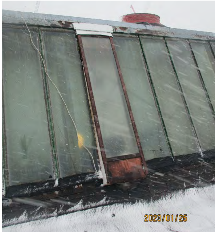
Close-up of a sawtooth skylight on the western portion of Building C. Note the fractured glass and sealants near the bottom of the frames. One window pane was altered with a new frame and appears to be crudely installed on the existing frame. The top flashing is rusted and appears to start deteriorating.
