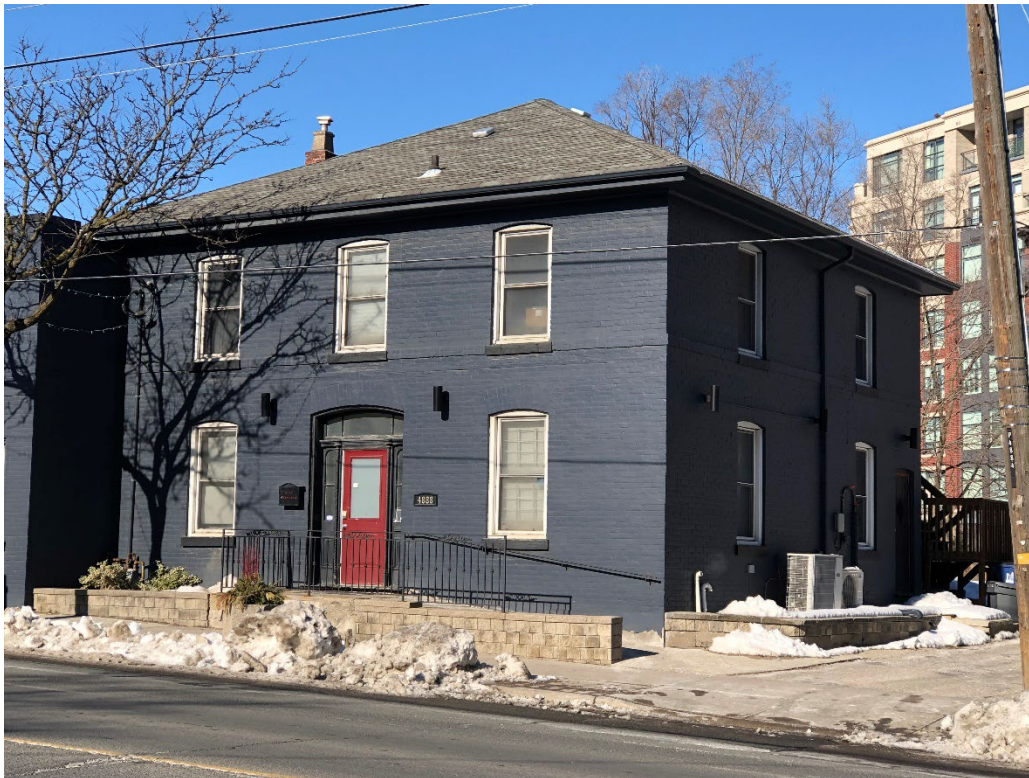
Figure 7: Oblique view of South (front) and East facades of 4888 Dundas Street West, 2023 (Heritage Planning)
