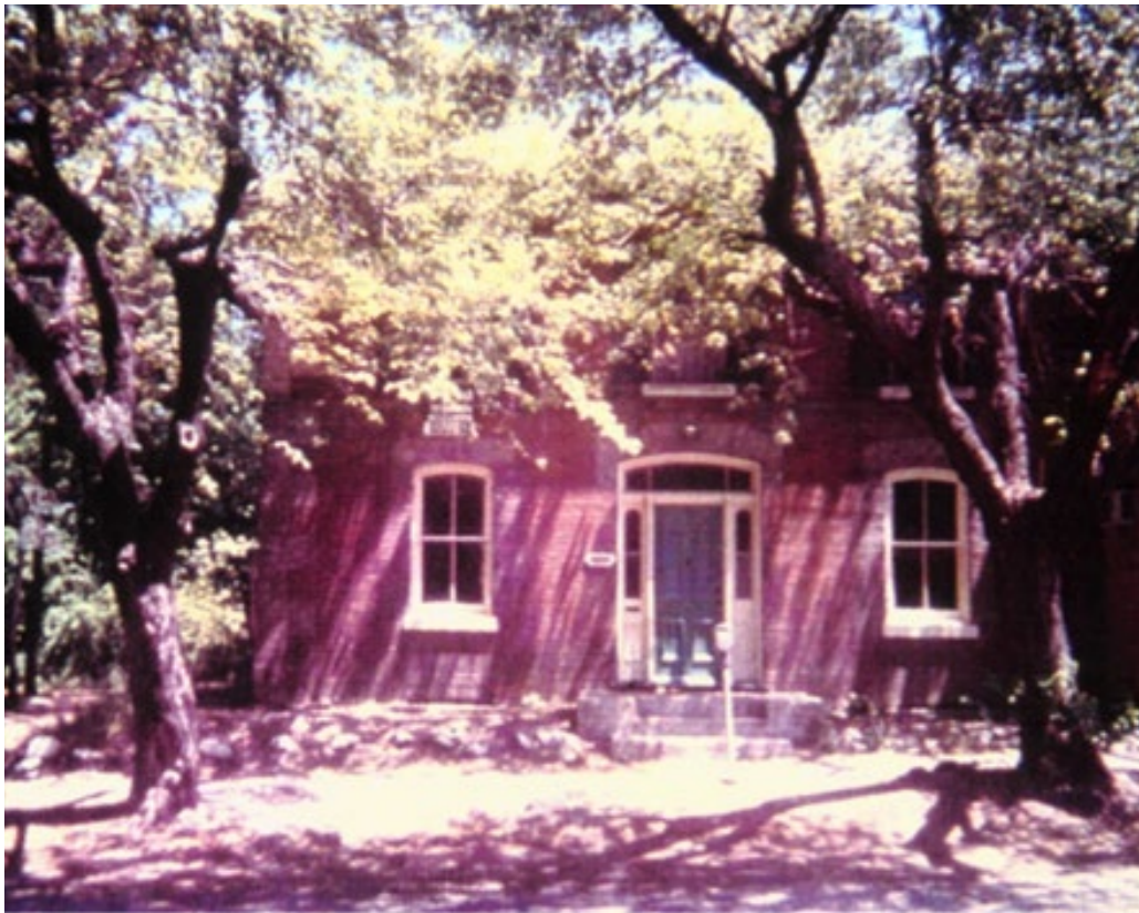
Figure 4: South (principal) façade of 4888 Dundas Street West, c. 1940s (Etobicoke Historical Society)
