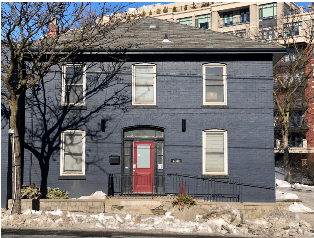
Figure 5: South (front) façade of 4888 Dundas Street West, 2023 (Heritage Planning)
