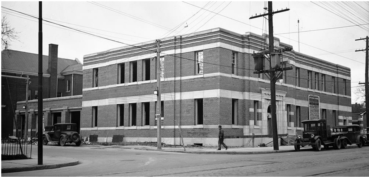
Figure 9: Image from December 1931, showing the new police station under construction (City of Toronto Archives; Fonds 200, Series 372, Subseries 1, Item 1071).
