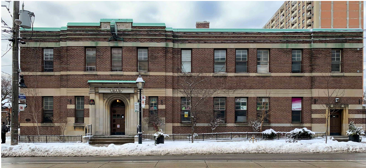
Figure 11: Principal (north) elevation of 1313 Queen Street West (Heritage Planning, 2023).
