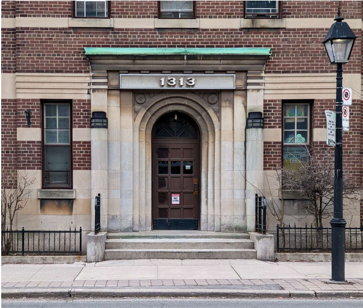
Figure 12: Main entrance, 1313 Queen Street West (Heritage Planning, 2022).
