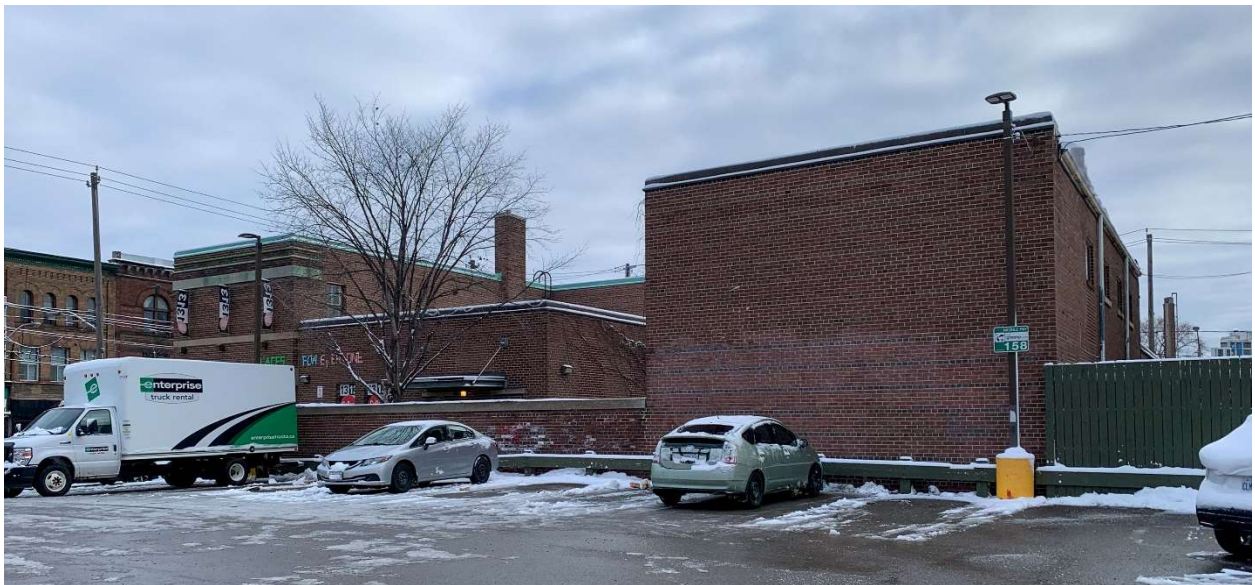
Figure 18: View of south and west elevations of 1313 Queen Street West from adjacent Green P parking lot (Heritage Planning, 2023).
