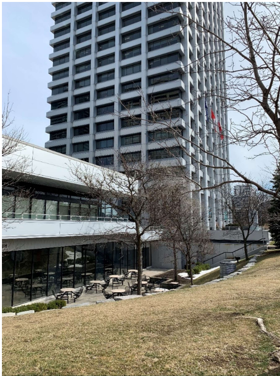
Figure 26. Two-storey building to the north of the Foresters tower, looking southeast, viewed from Don Mills Road, showing the sunken garden and landscape elements on the west side of the two-storey pavilion (Heritage Planning, 2023)
