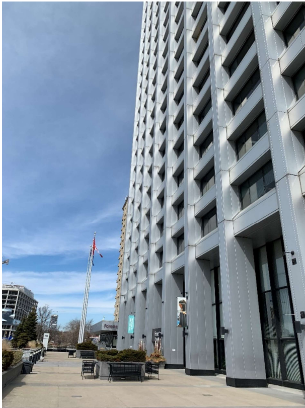
Figure 29. View of the west side of the raised public plaza, looking north, with planters and double-height first storey with massive piers (Heritage Planning, 2023)
