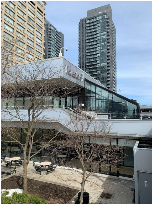
Figure 27. Two-storey pavilion (one storey is visible from the street) to the north of the Foresters tower, looking northeast, viewed from the raised plaza on the west side of the Foresters tower (Heritage Planning, 2023)
