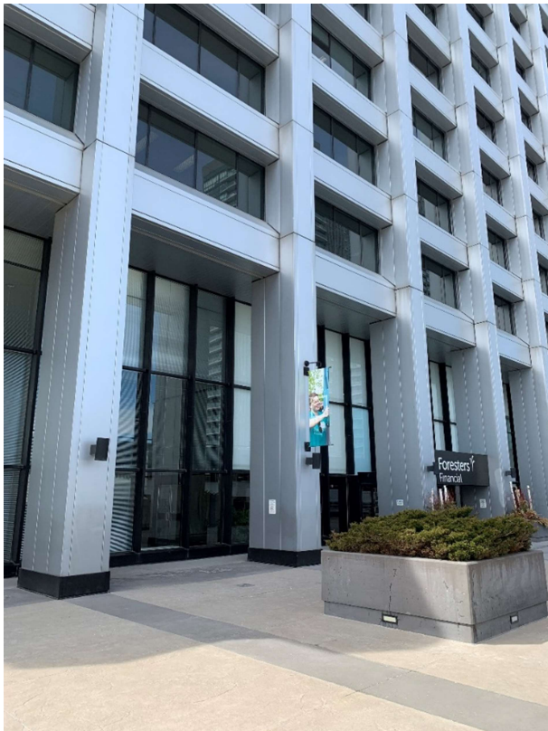
Figure 30. View of the east side of the raised public plaza, looking northwest, with planters and double-height first storey with massive piers (Heritage Planning, 2023)
