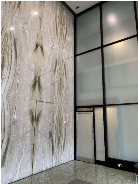
Figure 42. Inside the lobby of the Foresters tower, on the east side of the elevator core, looking north showing the book-matched marble wall panels with the hidden door (Heritage Planning, 2023)
