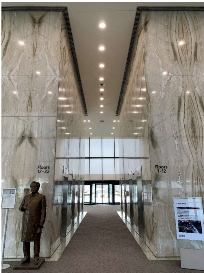
Figure 40. Inside the lobby of the Foresters tower looking west showing the elevator core with the book-matched marble wall panels creating a special pattern (Heritage Planning, 2023)
