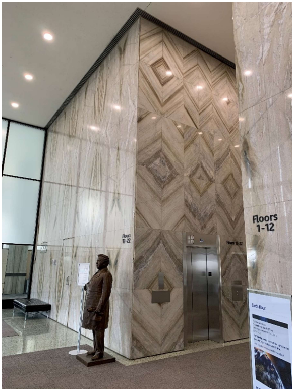
Figure 41. Inside the lobby of the Foresters tower, on the east side of the elevator core, looking south showing the elevator core with the book-matched marble wall panels creating a special pattern (Heritage Planning, 2023)
