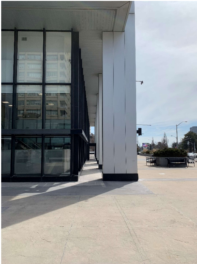
Figure 33. View of the northwest corner of the Foresters tower, looking south, showing the piers set forward from the elevation (Heritage Planning, 2023)
