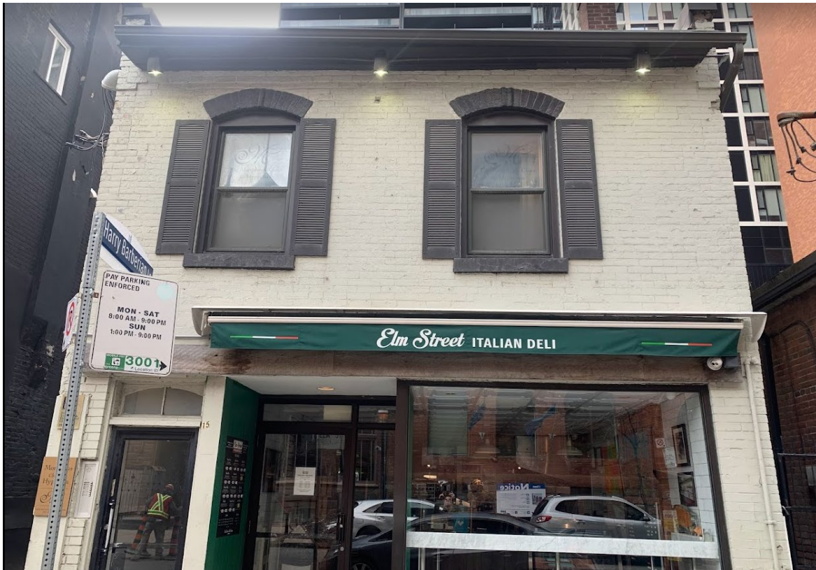
Image 15. Current photo showing the principal (north) elevation of 15 Elm Street (Heritage Planning, 2023)
