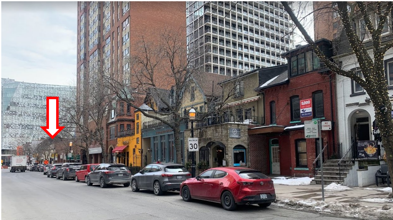
Image 25. Current contextual photo looking east along the south side of Elm Street and showing the collection of 19th century heritage properties located at 31-43 and 49 Elm Street. (Heritage Planning, 2023)
