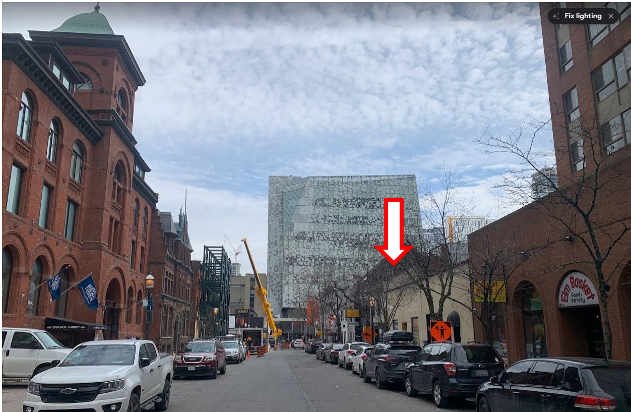
Image 23. Current contextual photo looking east on Elm toward Yonge and showing The Elmwood and The Arts and Letters Club (St. George's Hall) on the north side of the street directly across from the subject property. (Heritage Planning, 2023)
