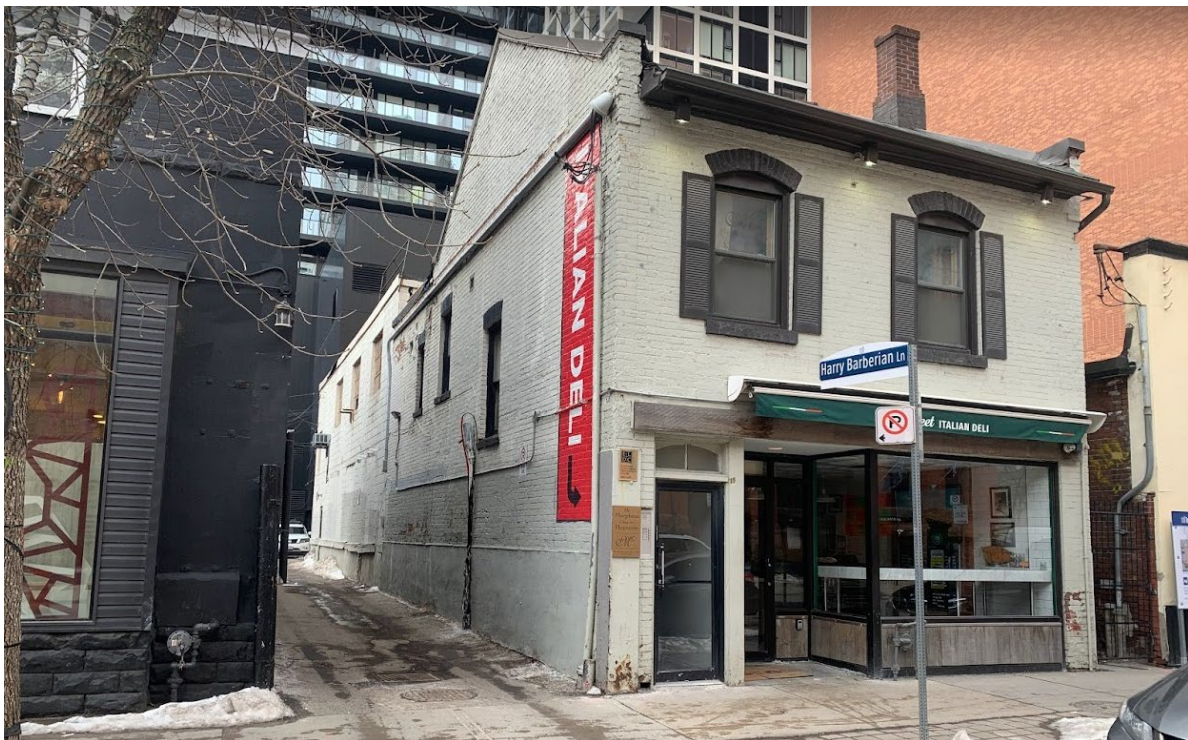
Image 18. Current photo looking south and showing the east elevation with rear concrete block additions completed by 1947 and adjacent to Harry Barberian Lane (Heritage Planning, 2023)
