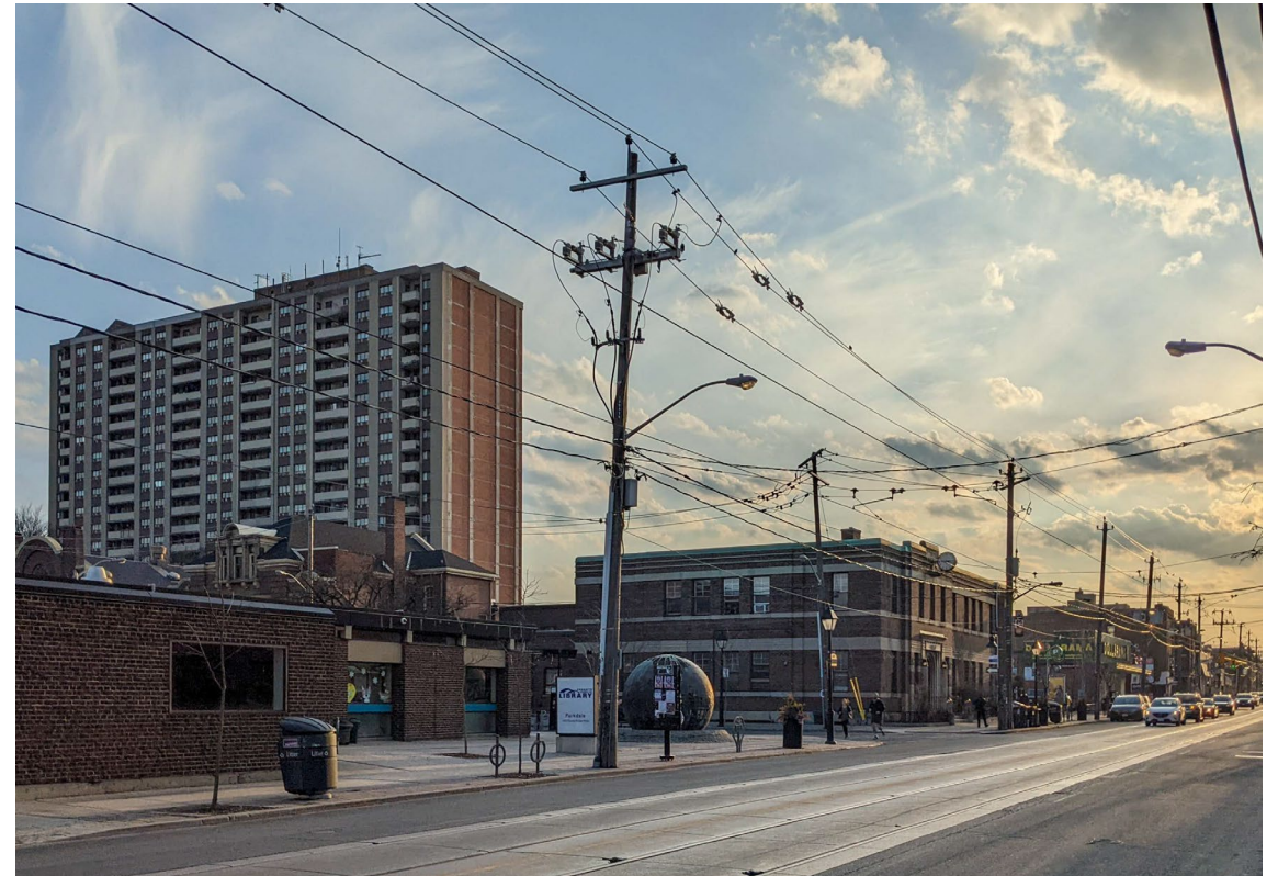
View southwest towards 1313 Queen Street West, operated by Artscape as the Parkdale Arts and Cultural Centre (Heritage Planning, 2022)
