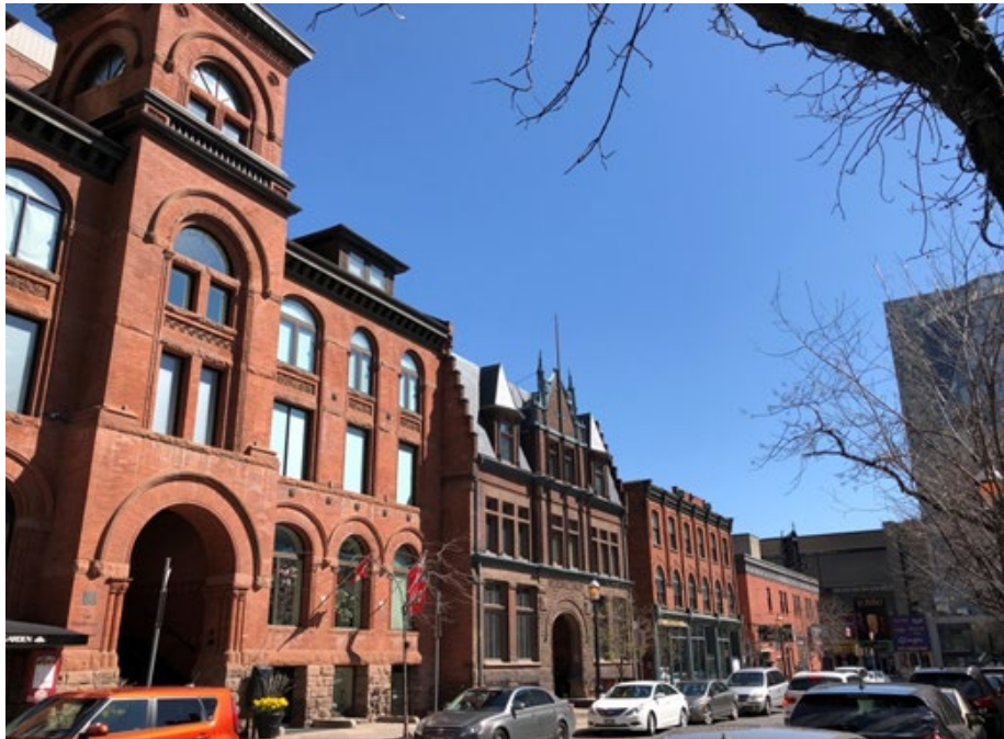
Current photo showing the collection of late-19th century heritage buildings located on the north side of Elm just west of Yonge, including (from left to right) the YWCA (now The Elmwood), St. George's Hall (now The Arts and Letters Club) and the James Fleming Buildings.
