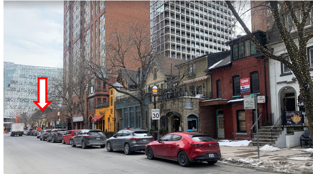
Contextual photo looking east along the south side of the street and showing the heritage properties located at 31-43 and 49 Elm Street, of which 15 Elm forms part of this 19 th -century collection of house-form buildings.
