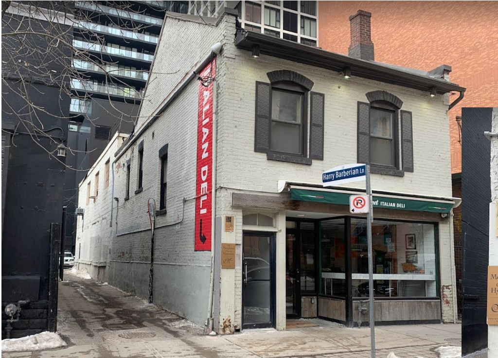
Looking south at the east elevation with rear concrete block additions completed by 1947 and adjacent to Harry Barberian Lane
