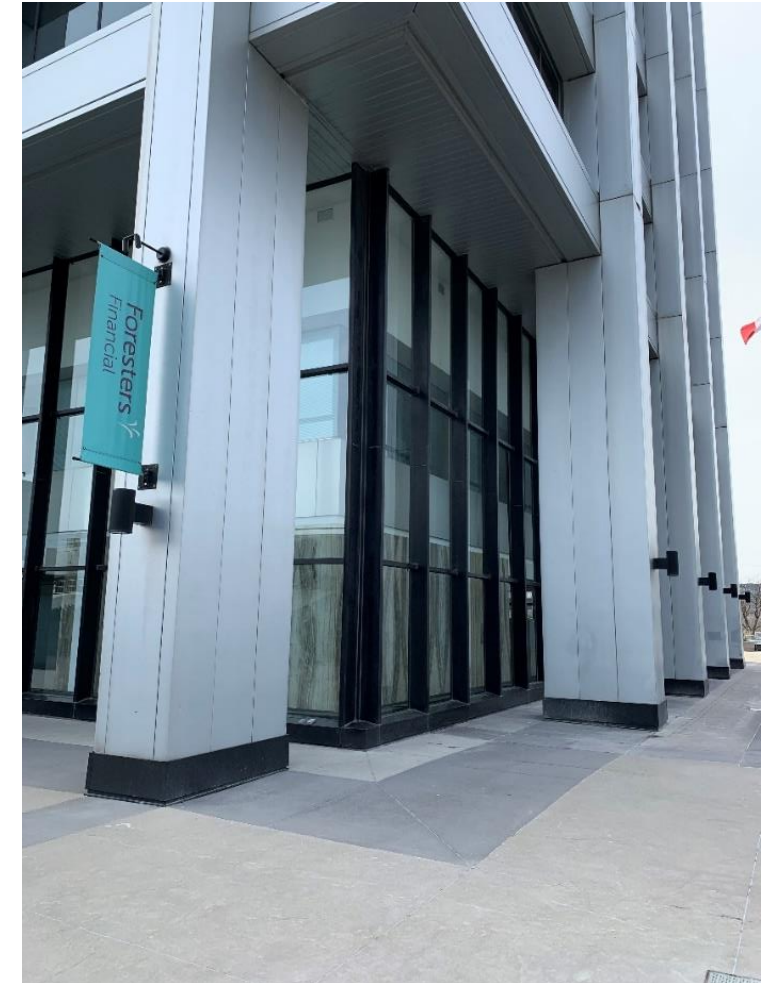
View of the north side of the raised plaza, looking west, showing the double-height curtain wall glazing at the first storey and the piers (Heritage Planning, 2023)
