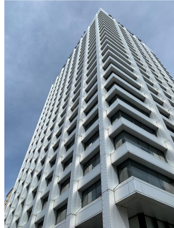
Southwest corner of the Foresters tower, looking northeast, showing the piers set forward from the elevation, ribbon windows, and the recessed chamfered horizontal panels beneath the windows (Heritage Planning, 2023)
