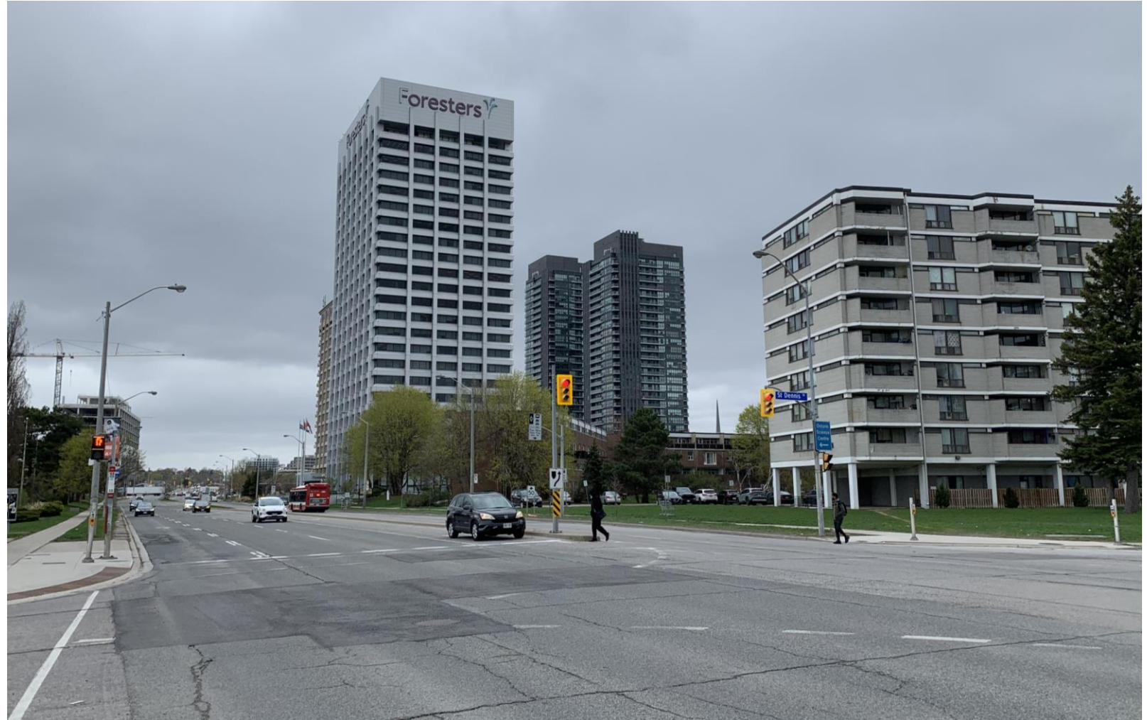
View of the south & west elevations of the Foresters tower, from southwest corner of Don Mills Road and St. Dennis Drive (Heritage Planning, 2023)
