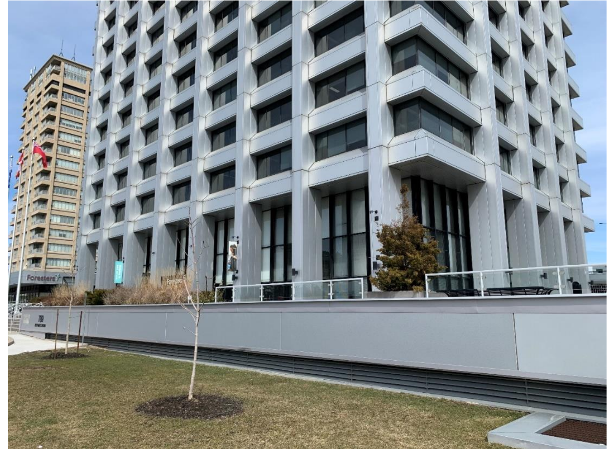
789-793 Don Mills Road: West side of the raised plaza, looking northeast, viewed from Don Mills Road (Heritage Planning, 2023)
